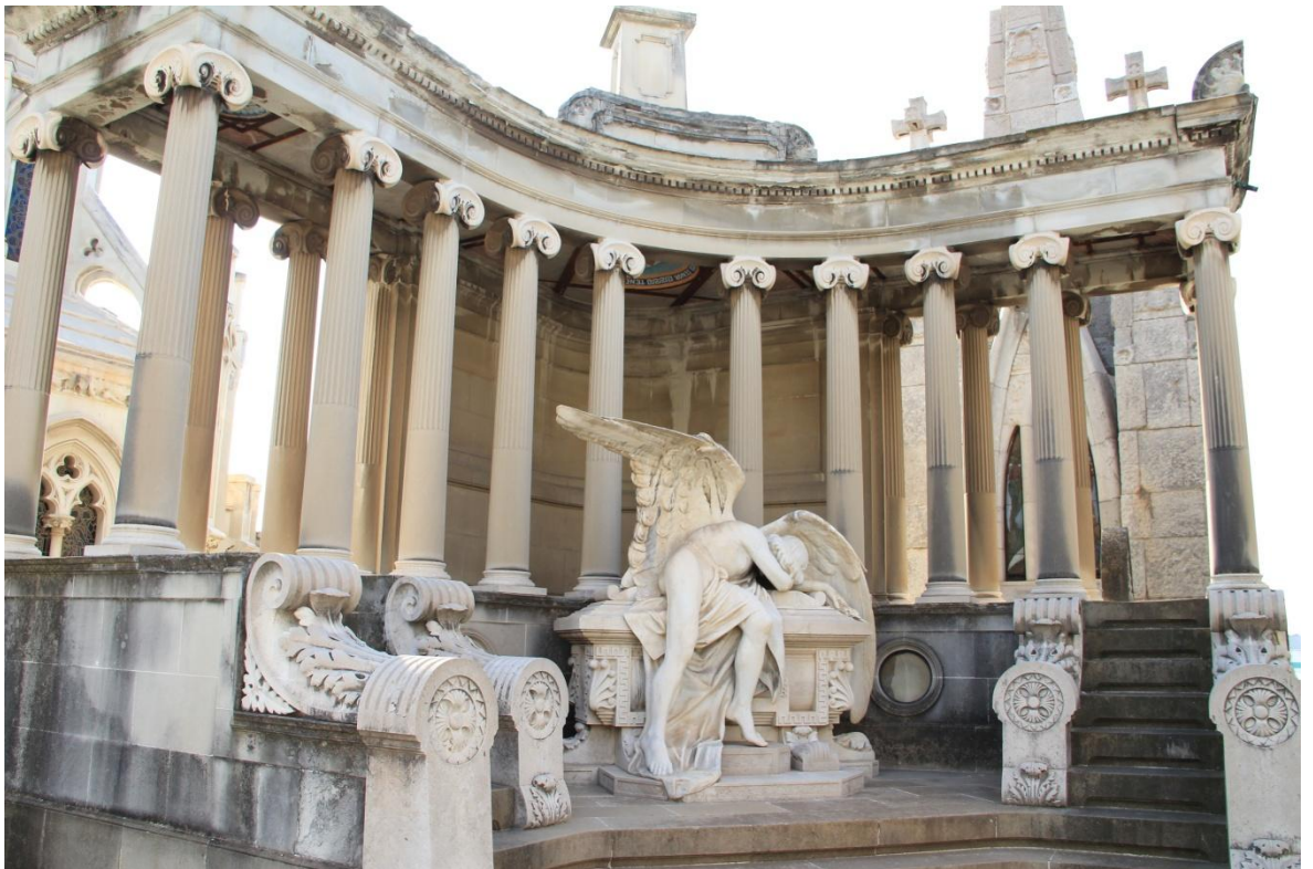
4.38. Antonio Vila Palmés (architect), Martínez and Fortuny (stone carvers), and José Campeny Santamaría? (sculptor, attrib.), Tomb commissioned by Augusto Urrutia Roldán, stone and marble, 1908-11, Montjuïc cemetery, Barcelona.
