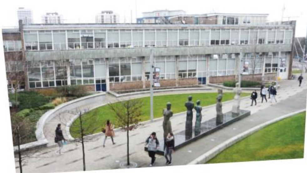
Figure 5 - 1 The Ellison Building at the University of Northumbria. Source: Author
