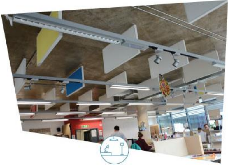
A5 - 45 Artificial Lighting and acoustics panels at the fifth year design studio in Plymouth University. Source: Author
