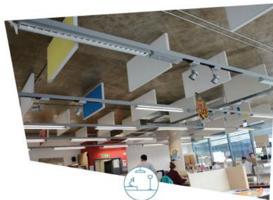
Figure 7 - 5 Artificial Lighting and acoustics panels at the fifth year design studio in Plymouth University. Source: Author
