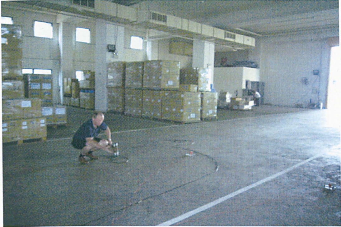
Figure 57 – Hammer testing of the floor bay
