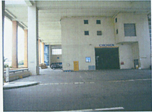
Figure 56b – View of the measured floor from the road
