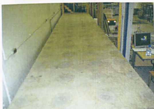
Figure 49a - RRF test structure
