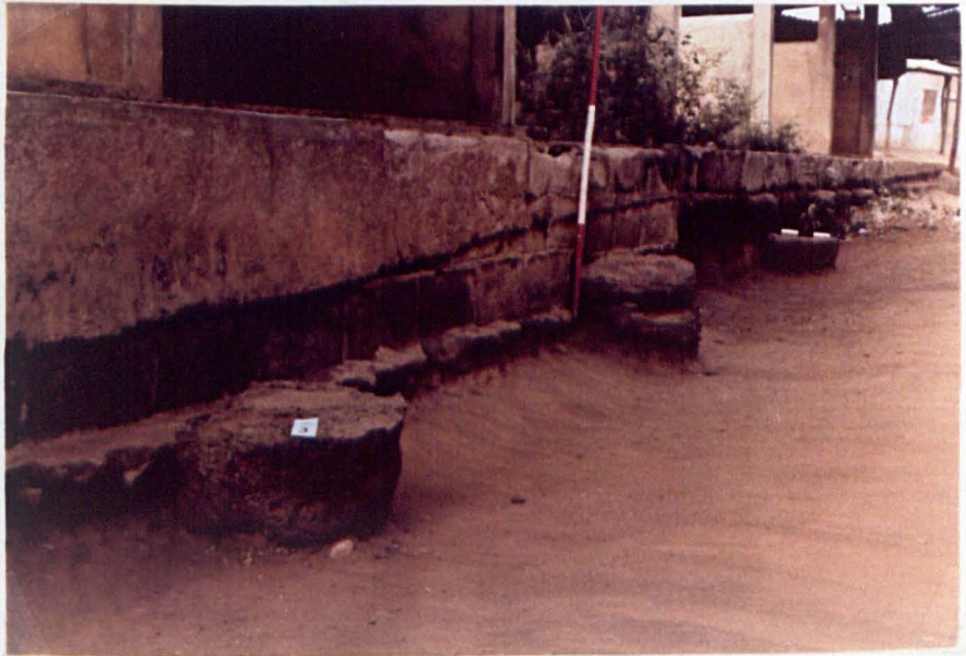
Plate 4:2 Slags used as building foundations.
