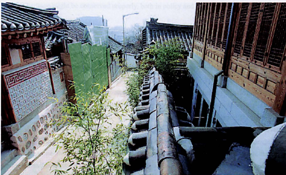
Fig.3.26 The first floor of the building is a concrete construction and the timber framed house rests atop; to the officials the traditional style tiled roof was the defining criteria upon which planning consent was given either (Source: Sin-jae Yoo, 'The Case of the Deformed Hanok', http://www.kahoidong.com/hank20070327e.html )
