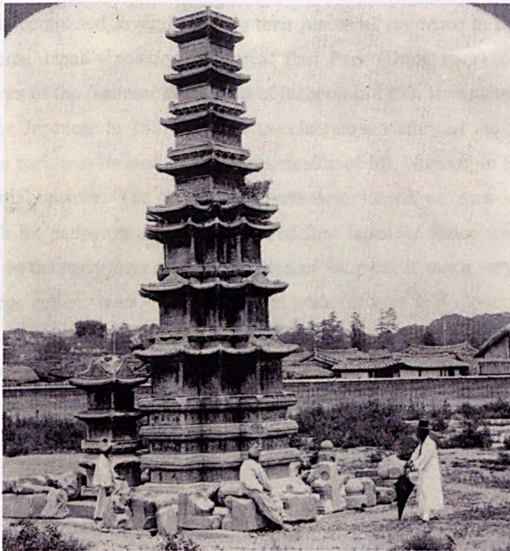
Fig. 2.65 Pagoda of Wongaksa Temple at Tapgol Park in 1904; commoners' houses were demolished, and once the site was flattened, it was enclosed with a brick wall. (Source: Won-mo Kim & Seong-gil Jeong (ed.), Korea 100 Years ago in Photographs (Seoul: Catholic Pub., 1986), p. 100.)
