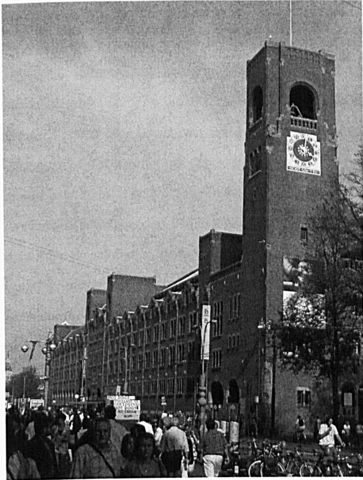
Figure 1.6 Amsterdam Exchange Building, Netherlands, 1897-1903, by Hendrik Berlage.
