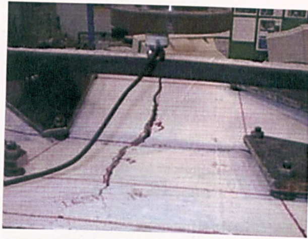
Figure 3.20: Transverse crack in Test 16.
