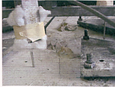
Figure 5.7: Development of transverse crack in Test 4.
