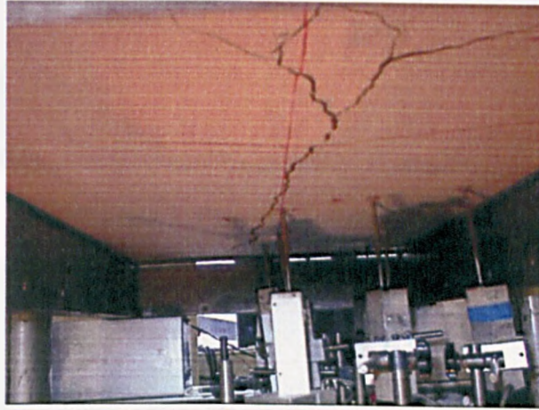
Figure 3.16: Formation of diagonal cracks with increasing load.
