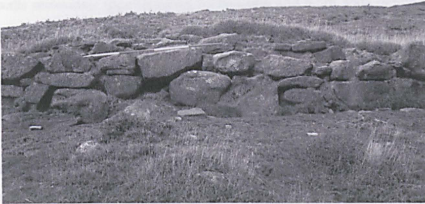
Photograph 5.2. Dovestone Clough settlement platform revetment
