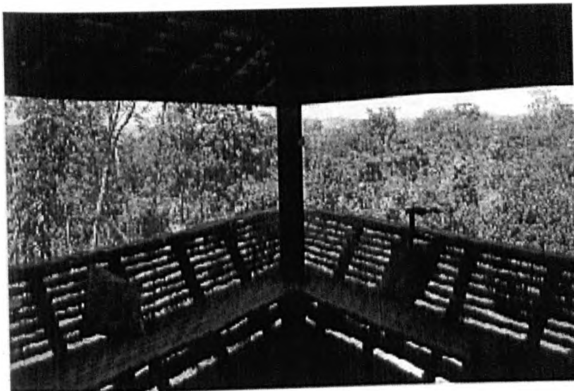
Figure 3.14 The Malay anjung — a timber veranda raised on tall, slender columns and used as an outdoor extension of living area. The Salinger House, Bangi, Selangor, Malaysia. Architect: Jimmy C S Lim. (After Powell 1998)
