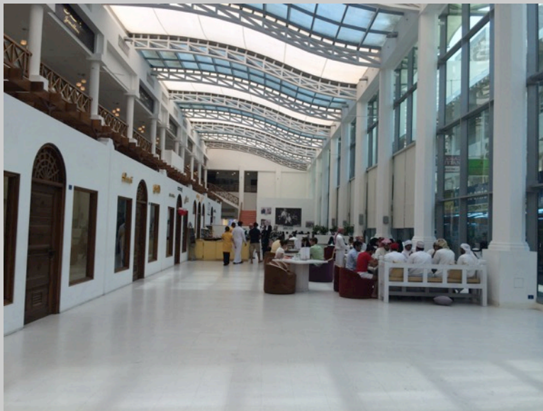
Figure 5.15 The Atrium in the mall acts as attraction point for middle class users to Bab Al-Bahrain Area.
