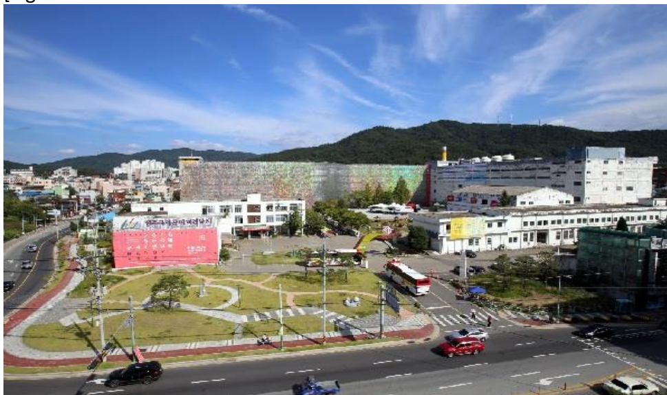
[Figure 8-1: Cultural Facilities and the Main Venues of CCEA in Naedeok-dong]
