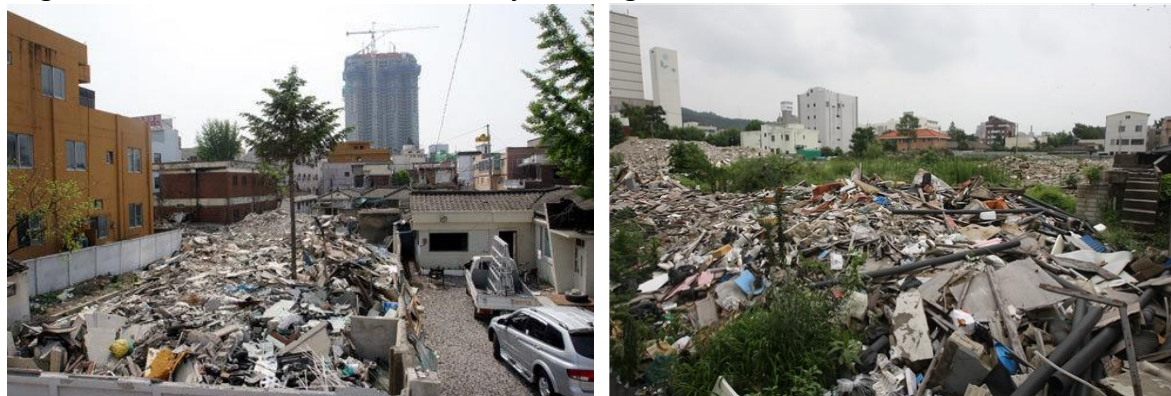
[Figure 6-7: The Demolished Area of Sajik 4 dong]
