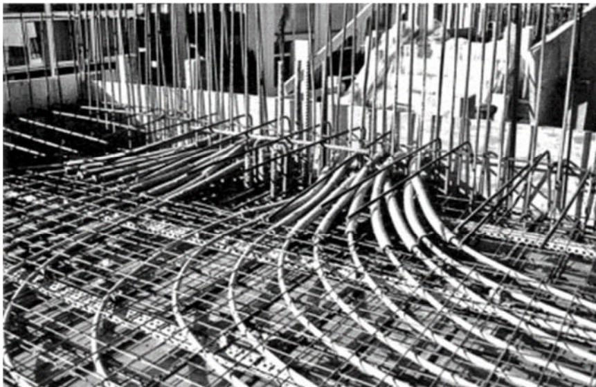
Figure 2.10 : Absorber pipes entering a concrete slab (Brandl, 2006)
