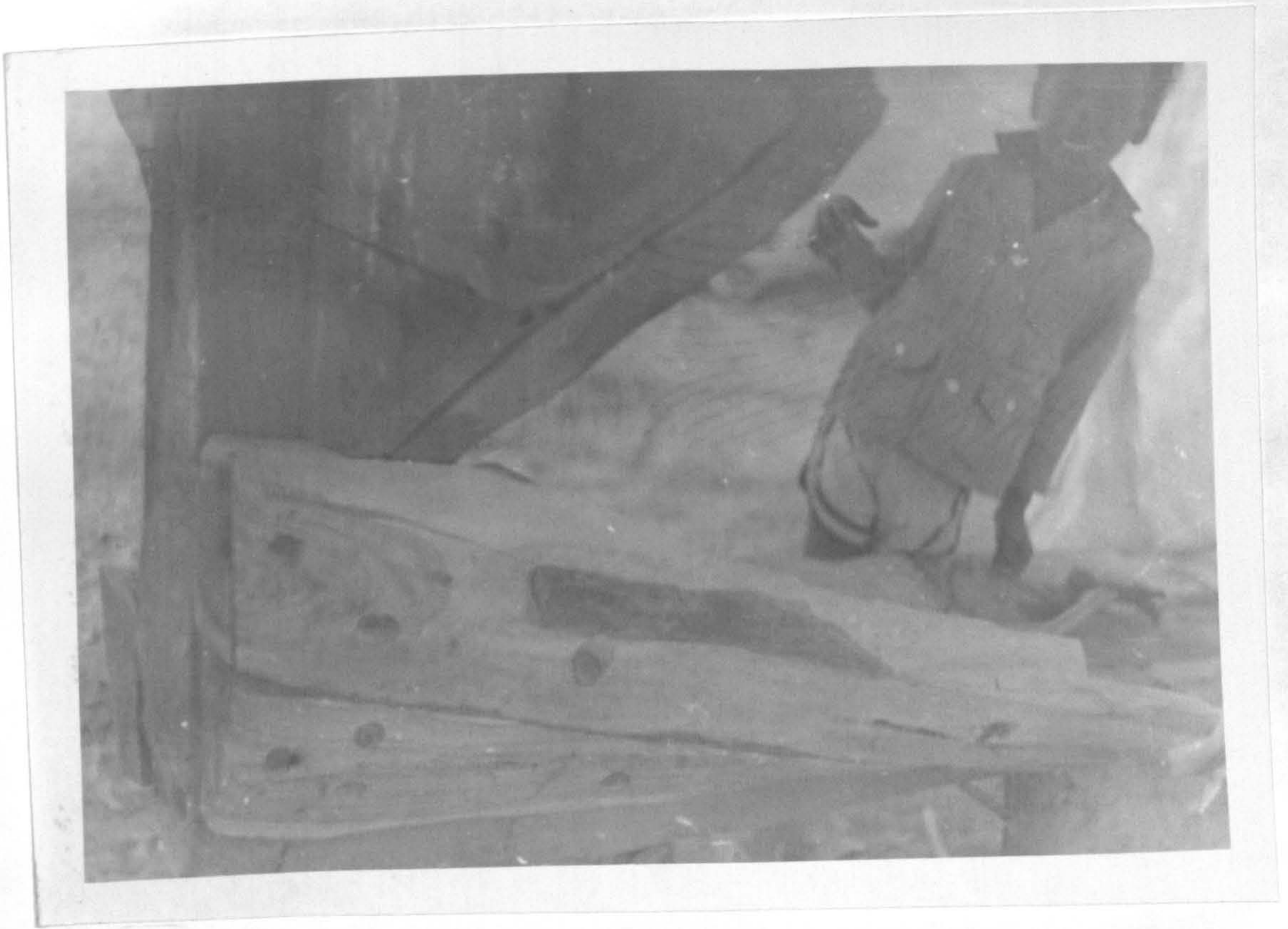
Plate 8. The lowermost planks spiked to the sides of the keel and the bottom of the stern post.
