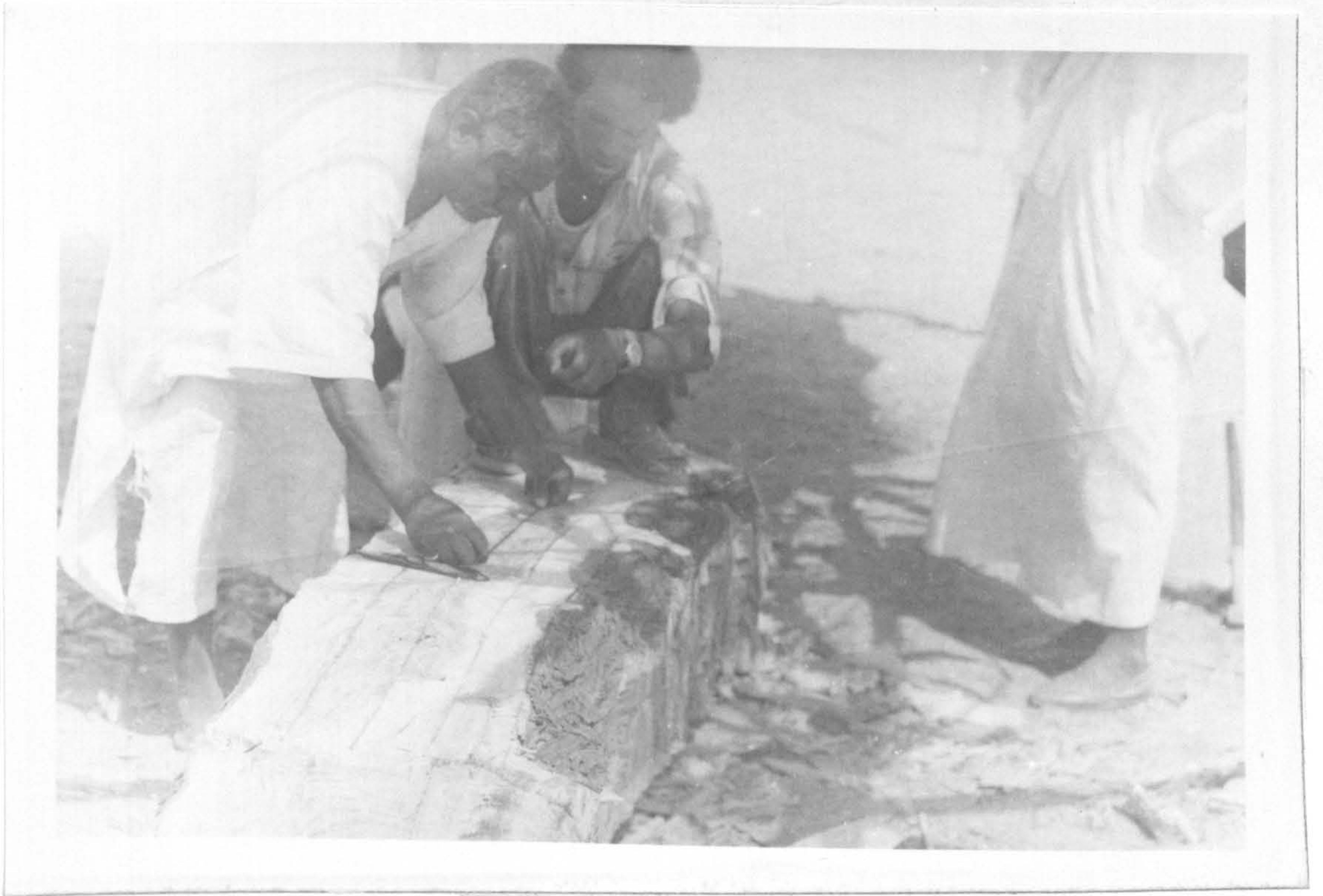
Plate 3. The master craftsman marking the curvature and width of the planks using a string dipped in black paint.
