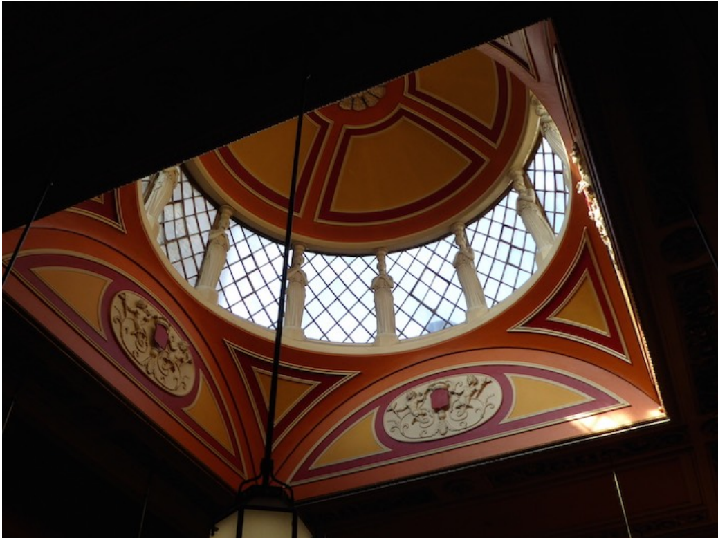
Charles Augustin Busby, Commercial Rooms, Bristol, 1809-11. Photo: Philip Wilkinson.
