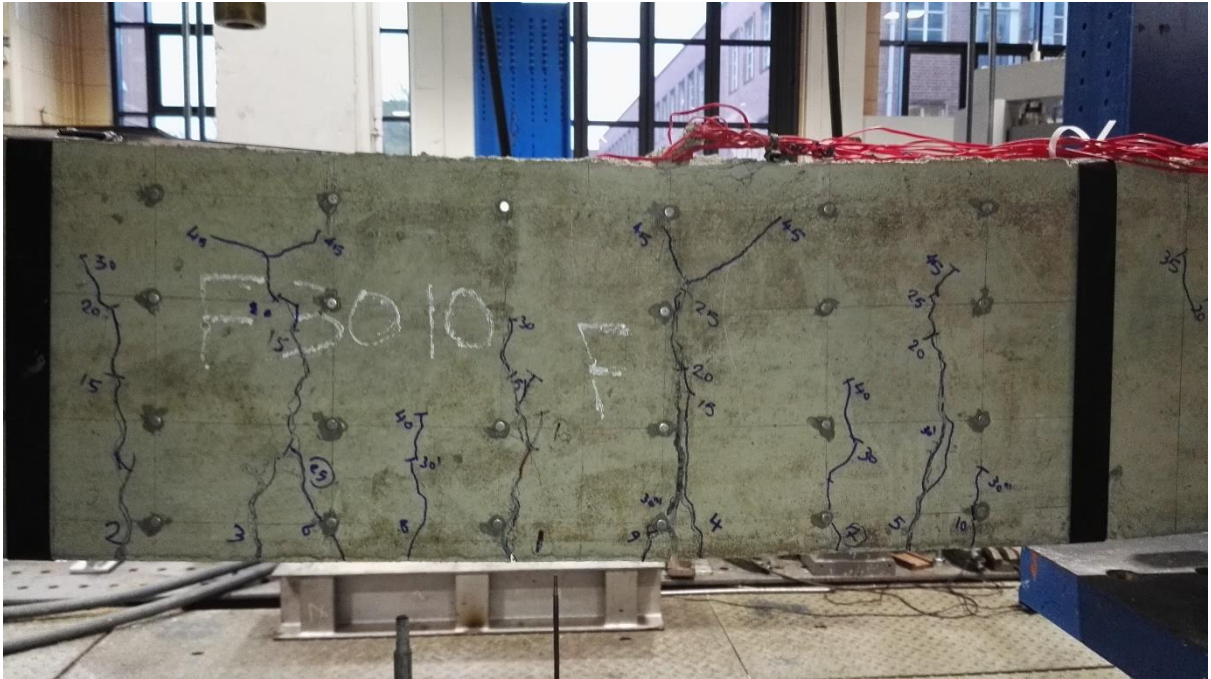
Figure C.10 Final cracking pattern in constant moment zone in beam B3010.
