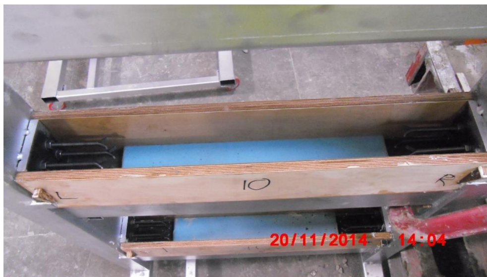
Figure A.2 Restraining frame before casting (inside mould).
