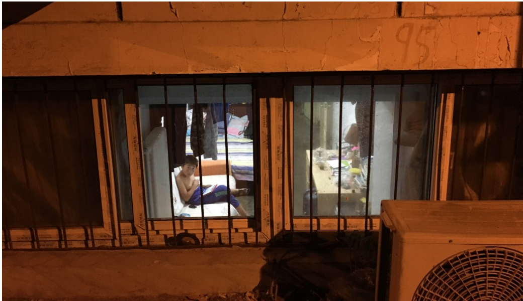
Photo 9-28 Semi-basement with window
