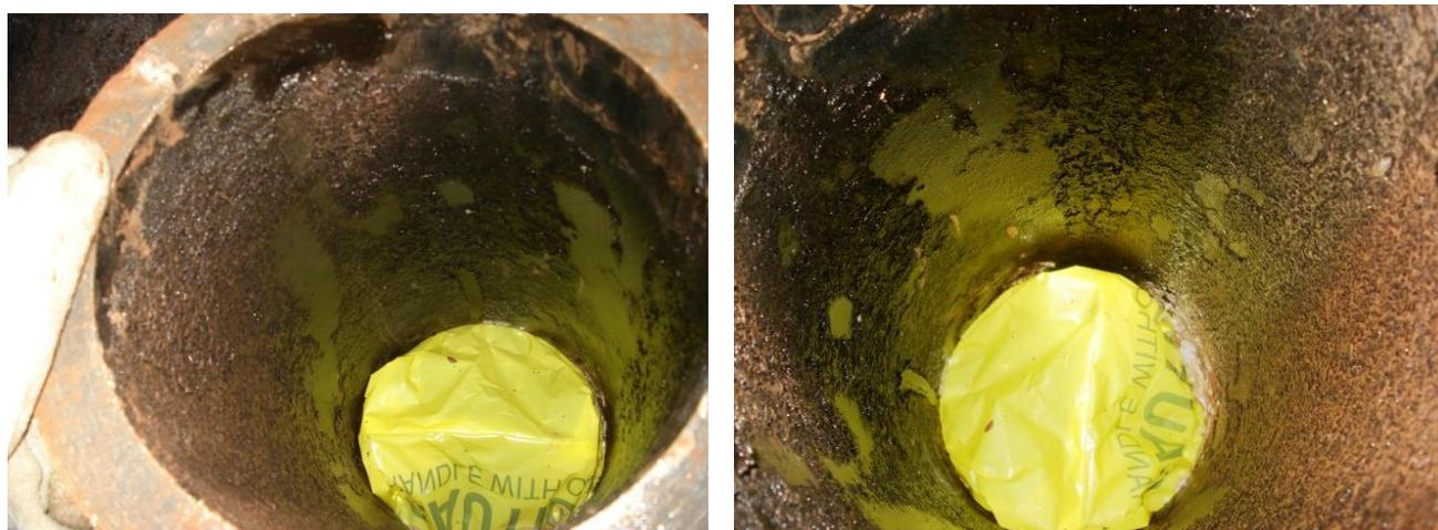
*Figure 29: Pre-cleaning intervention pipe cut out*
