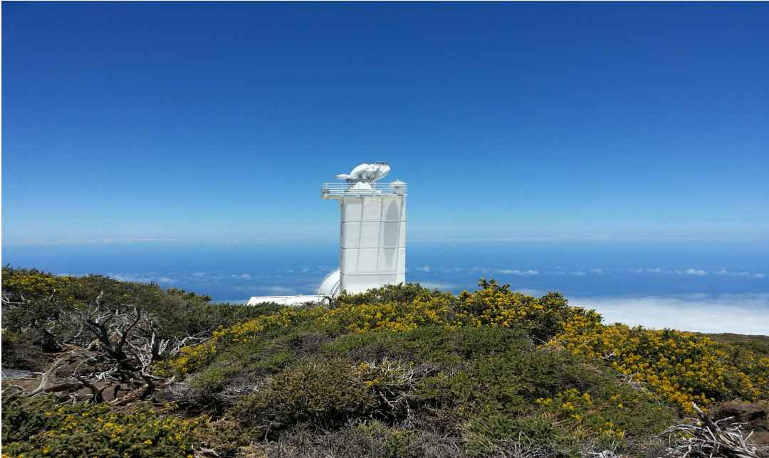
(a) The Swedish Solar Telescope (SST) at the island of La Palma, Canary Islands. The primary mirror of the telescope can be seen at the top of the tower building. The building structure itself harbors the vacuum tower beneath it. (Image courtesy: Nabil Freij.)
