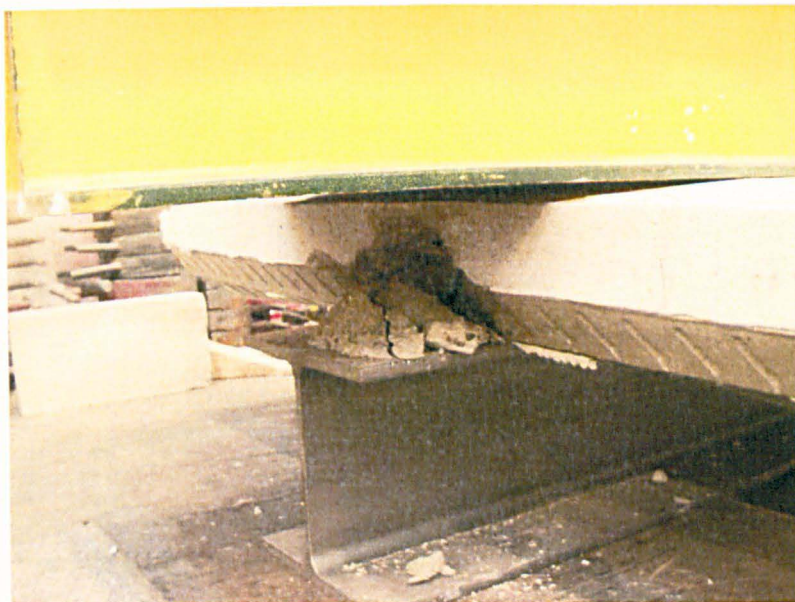
Figure 3.31 Concrete spalling at free end of specimen PTSN 1-1
