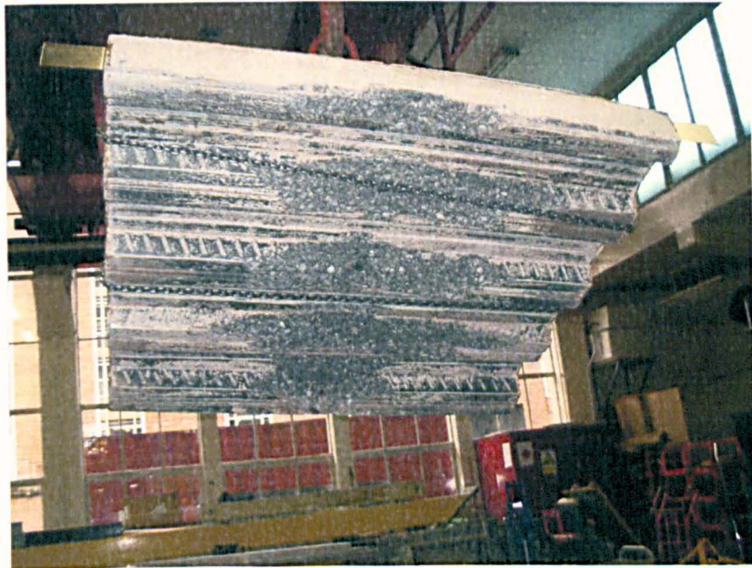
Figure 3.19 Underside of the slab of test PTS 2-1 showing pull-out failure surfaces
