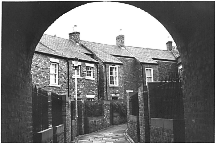
15.17 Backyard of The Island Block - an excellent example of how to treat a small backyard.
