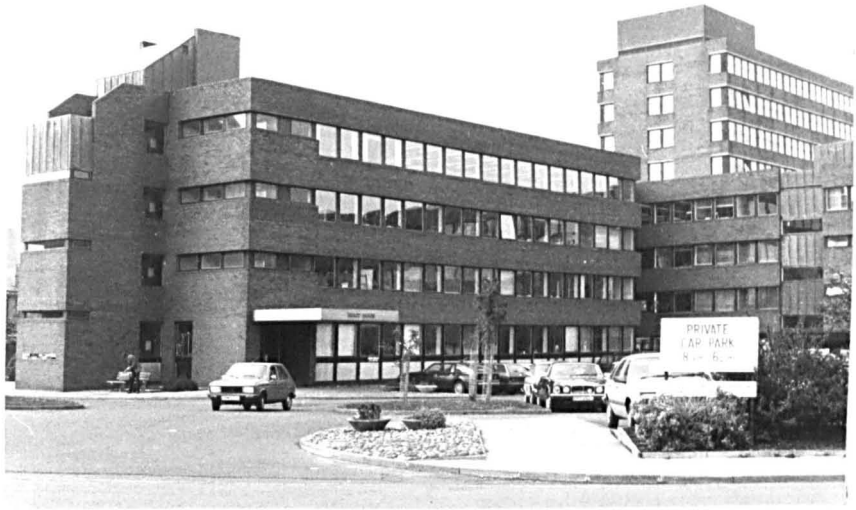
15.01 North Housing Association. Head office in Regent Centre, Gosforth.
