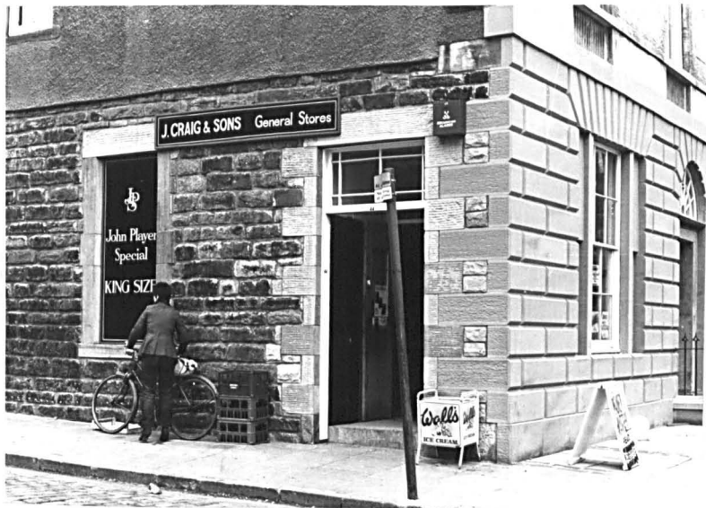
14.06 The shop at the corner of Graham Street. The shop owner had one of the former shops, projecting from the Lauriston Place facade, and refused to move. A compromise was reached, and he moved into this corner shop, which is now very prosperous.
