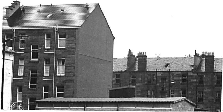
13.07 Before and after renovation. Note the new windows and the removal of the chimney stacks which considerably changes the appearance of the buildings.
