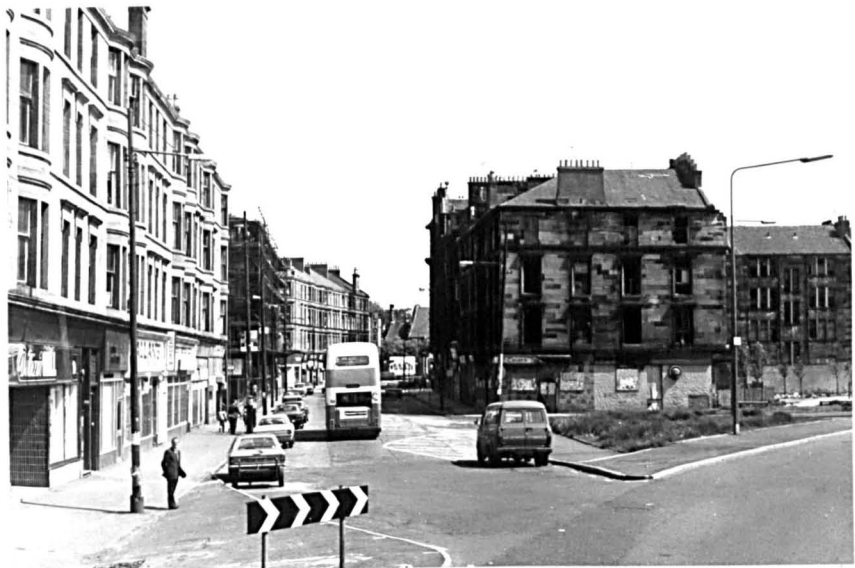
13.02 'Entrance' to Govan. The ringroad continues to the right; the house in front is unfortunately going to be demolished.
