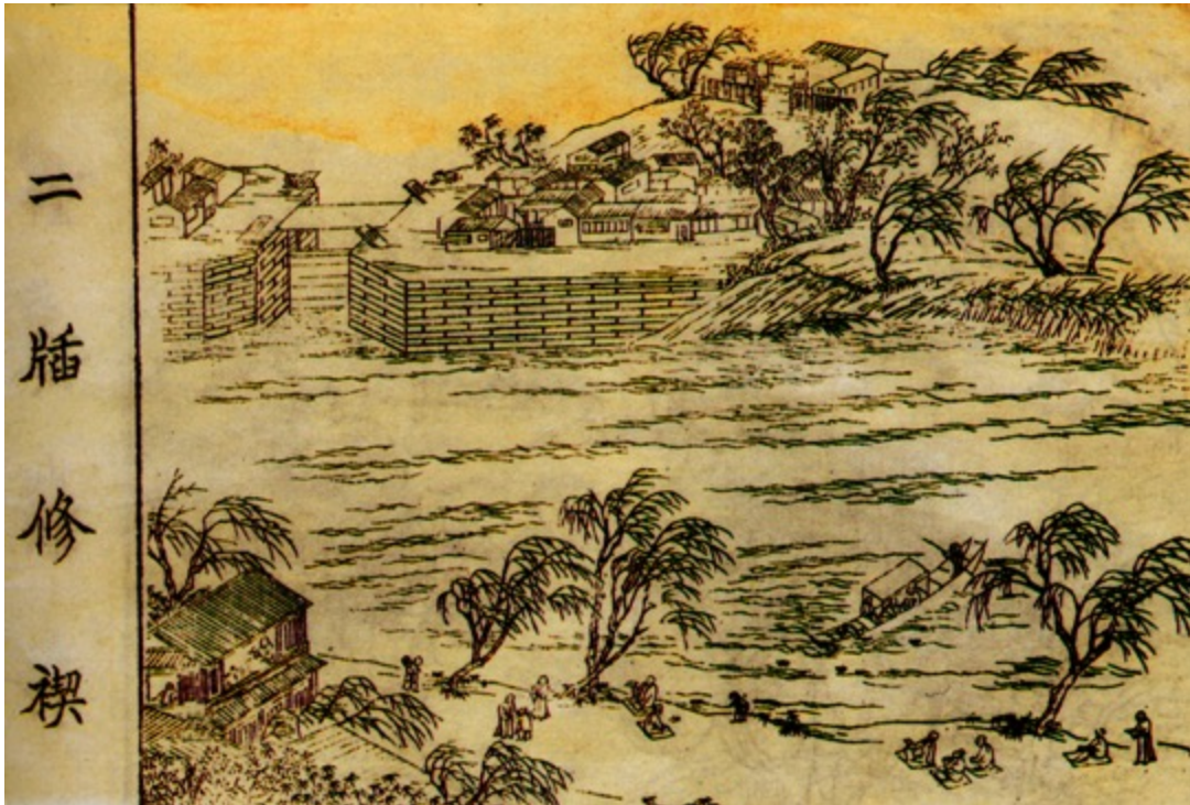
Figure 4.10 The Qingfeng Lock on the Tong Hui River. It is a typical canal lock which shows their basic structure. Some materials, such as stone slabs and beams, can also be seen. There is a bridge over the lock gate, a movable one which could be removed when barges were going through the lock. The surrounding landscape including earth bank, residential houses, a two-store pavilion and willow trees are also shown. Source: Liao Cheng Canal Museum. The sketch was originally from Linqing's Hong Xue Yin Yuan Tu Ji (Illustrated Traces of a Life) from the early nineteenth century.
