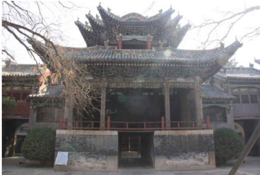
Figure 6. 13 These two photographs of Shan Shan Hui Guan (Shanxi and Shaanxi Provincial Guild Halls) in Liao Cheng city show the threshold and the performing stage in the eastern corner of the courtyard. The roof of the threshold is of the hip-and-gable roof style, with the words Shan Shan Hui Guan written on the top of the main gate. There are also the words lv zhong and dao he on top of the side gates, which represent the business faith of the native merchants. 749 In 1743, when merchants from Shanxi and Shaanxi started raising money to build a base for themselves to ‘worship their god (guan di) and remember their homeland’, the guild hall was built on the western bank of the Liao Cheng section of the canal. 750 According to the inscriptional records, the material and craftsmen were both transported from their region of origin in order to fully represent native architectural characteristics. Source: photographs taken by author in winter 2014.
