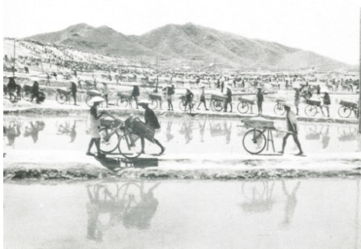
Figure 5.20 The photo shows large numbers of wheelbarrows being used to carry earth. The wheelbarrows here might have been ‘upgraded’ with the installation of bicycle wheels, as the wheels look larger than usual.
