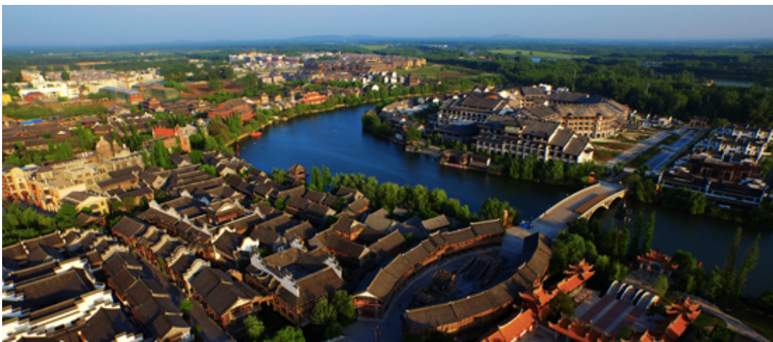
Figure 6.27 This aerial photo shows the inharmonious relationship between the newly built replica town area and the original town area. The guidelines in the Washington Charter say, ‘the conservation plan should aim at ensuring a harmonious relationship between the historical urban area and the town as a whole’. Source: Yan Yu (photographer), ‘zhou you qi lu man you tai’er Zhuang (travel around Qilu and Tai’er Zhuang)’, The People’s Website (2015): < http://tour.dzwww.com/lvnews/201505/t20150512_12365457.htm > [accessed 10 th
