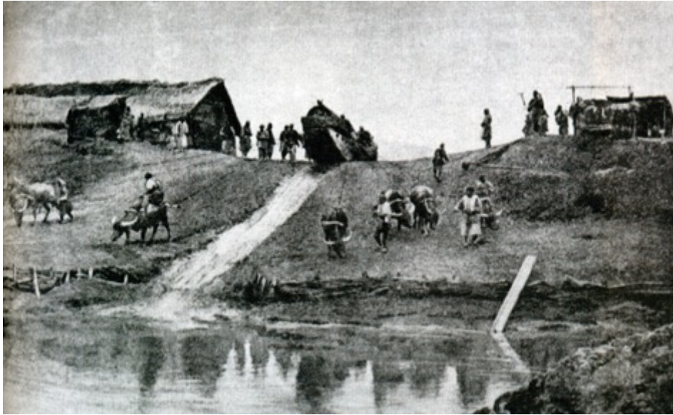
Figure 2. 7 An early twentieth century picture shows a barge being pulled over a double slipway by ox. Source: Liaocheng Canal Museum.
