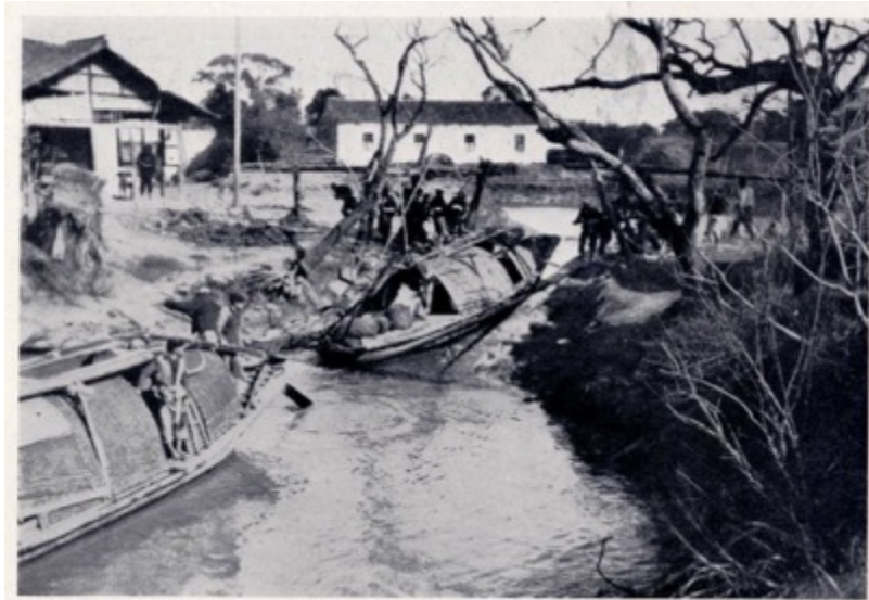
Figure 2. 8 A photo taken in 1926 shows that double slipways were still in use at that time. Source: Liaocheng Canal Museum.
