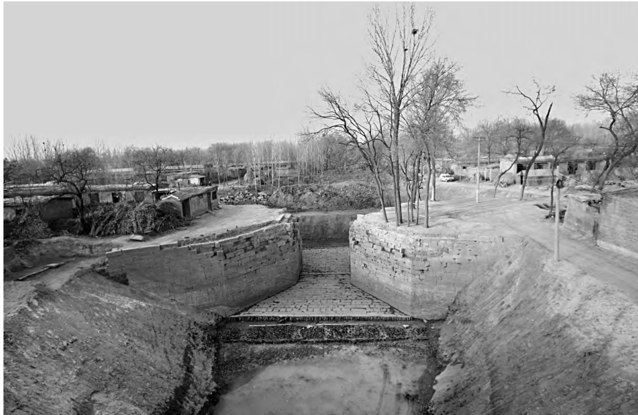
Figure 6.5 The southern side of the Tu Qiao lock when it was discovered in 2010 during the investigation of the south-north water transfer project. The layer of stonework under the lock gate can be seen, as well as the general structure of the lock. Because of the disused waterway and lock, the residential houses have expanded to the bank. Source: Liao Cheng Institute of Cultural Relic Archeology, Liao Cheng Cultural Relic Bureau and Administration Office of Cultural Relic, Dong Chang District, Liao Cheng, p. 40.
