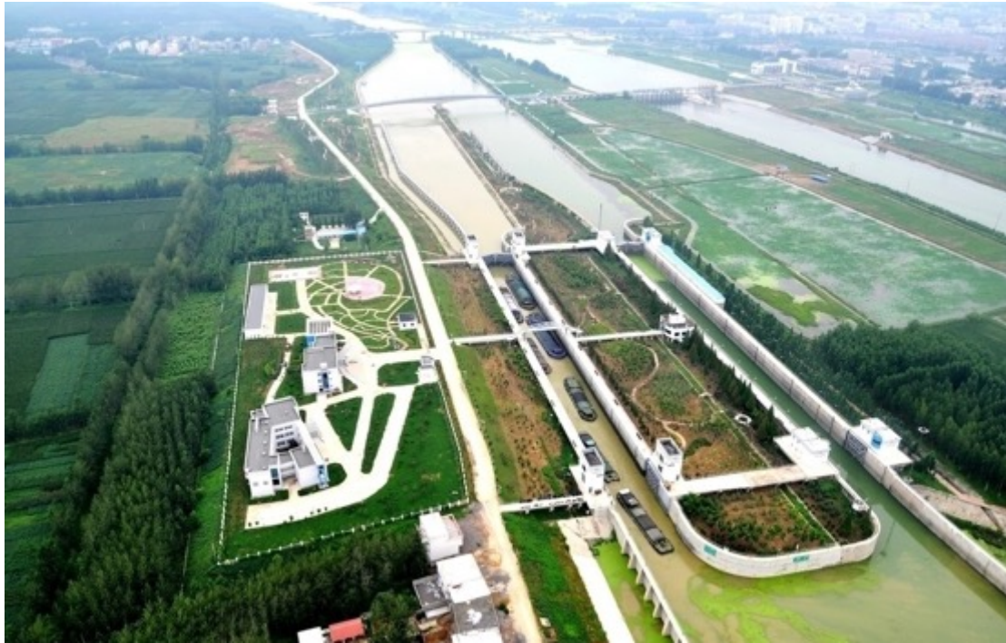
Figure 5. 26 An arial view of the Tai'er Zhuang lock, which shows the upgraded modern embankment and lock. Source: 'Aerial Photographs of the Tai'er Zhuang Lock', Ni-pic Web (2012) < http://www.nipic.com/show/-1/49/6210068ka9faf9fd.html > [accessed 23rd May 2016]
