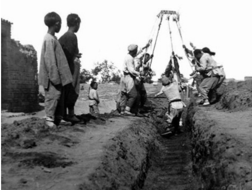
Figure 4.18 This photograph was taken in the 1930s and shows that the same way of compacting earth was still used in the early twentieth century. Source: Liaocheng Canal Museum. Photograph taken by William Smith.
