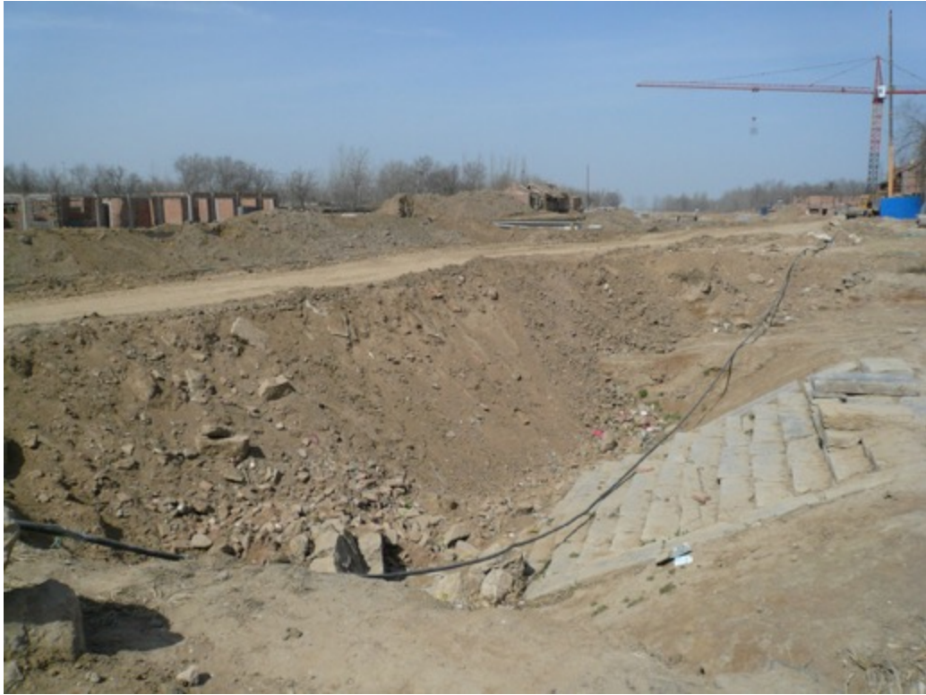
Figure 6.33 The photo taken by author shows part of the excavated Qi Ji dock in 2013. The stairs were left uncovered after it was excavated, and no evidence of any protection measures could be found.
