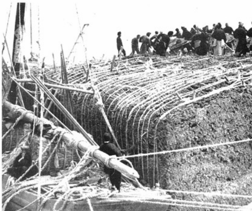
Figure 5.5 photo shows how the kaoliang stalks structure were lowered into a dyke breach. The spar used to attach the ropes of the structure can be seen on the large boat. Source: Needham, PLATE 383.
