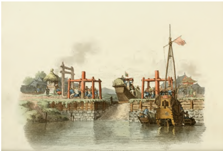
Figure 2. 6 An early nineteenth century painting shows a canal barge passing over the double slipway. It also shows the structures on both sides of the slipway, which were made of stones and timber. Source: Alexander William, 'Front View of a Boat, Passing over an Inclined Plane or Glacis', in The Costume Of China: Illustrated In Forty-eight Coloured Engravings (London: William Miller, 1805)
