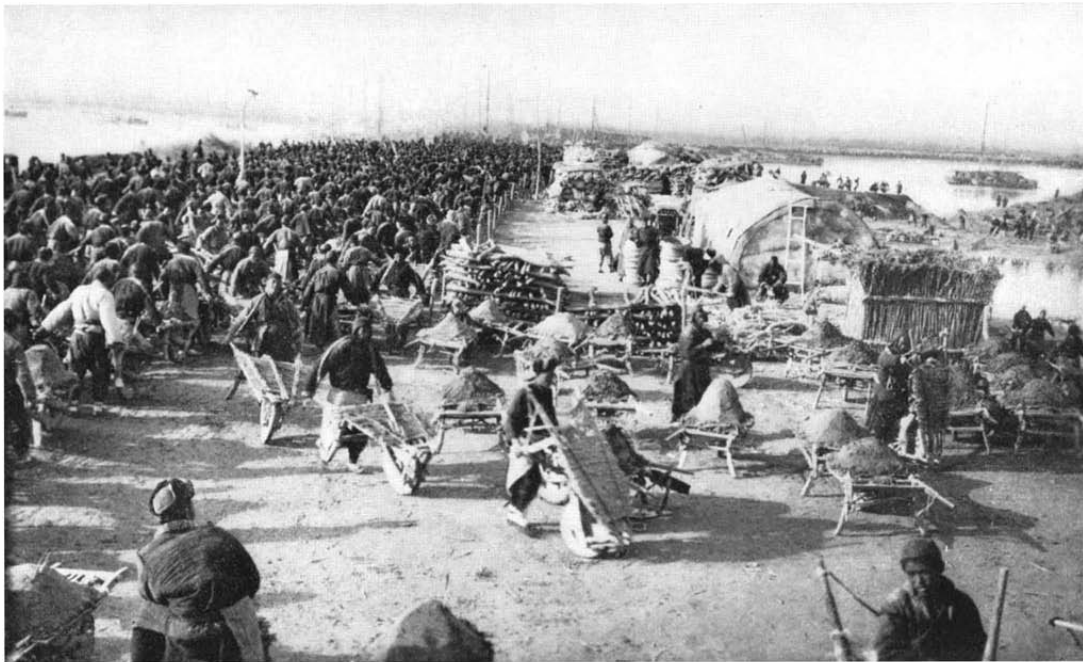
Figure 5.12 The photo by Todd shows the busy scene of the site half a mile away from the working point: numerous men are carrying supplies using wheelbarrows on the left, and on the water side we can see some tied kaoliang stalks. This photo shows a typical scene of a water control project in which most of the work was relied on manpower. This project involved about 25,000 men working at the same time, in winter, of which the hardship can be imagined. Source: Todd, p. 5.
