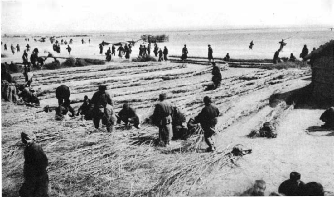
Figure 5.7 The photo shows men making the willow fascines on an open yard, to use in the 'stone sausage' structure. Source: Todd, p. 7.
