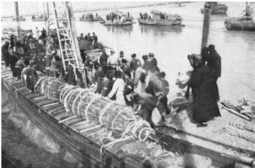
Figure 5.8 photo shows one giant 'stone sausage' being moved to a boat, where the men are preparing to place it into the water. Source: Todd, p. 8.
