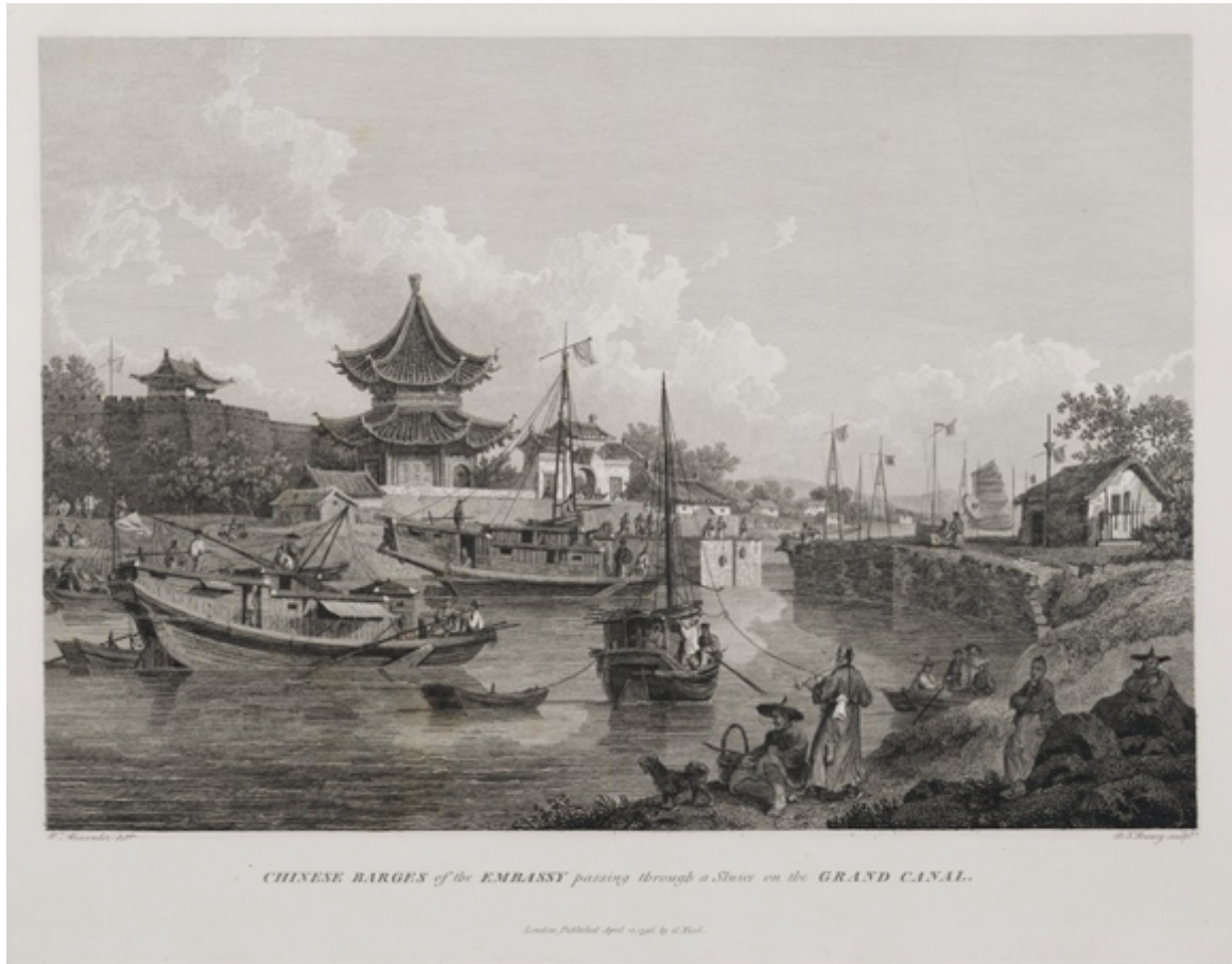
Figure 4.11 This painting from the late eighteenth century shows a scene of the barges of a British embassy passing through a lock on the Grand Canal. We could see the groove on the lock, designed to keep the lock gate's wooden beams in place; here they have already been lifted up. There are also many other elements in the picture, including the earth bank, plants, the lock keeper's cottage (right) on the side of the lock, and the more majestic tower behind the threshold (left) which was a wei suo (guard post) for the troops stationed along the canal. The people sitting on the bank might be trackers waiting for business. Source: Yale University Library, Beinecke Rare Book and Manuscript Library, originally from An Authentic Account of an Embassy from the King of Great Britain to the Emperor of China .
