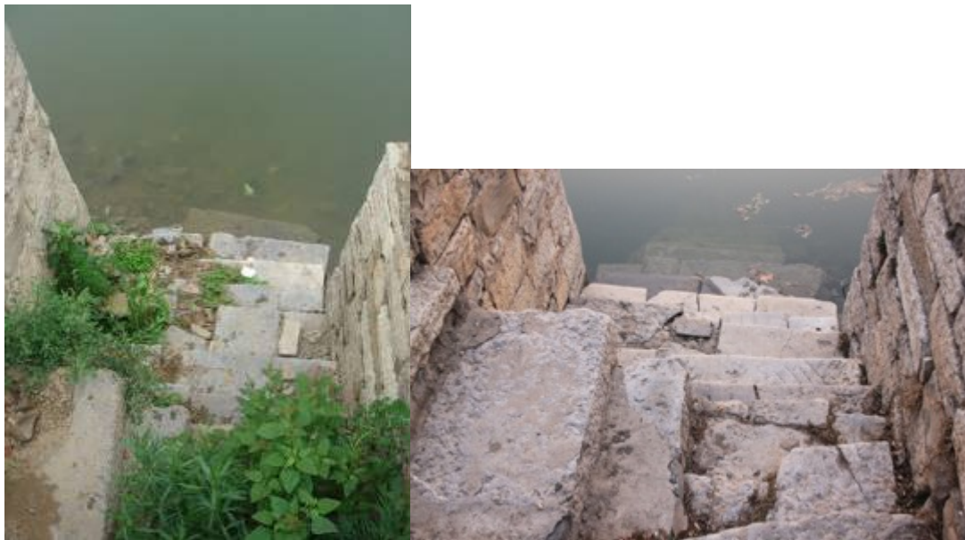
Figure 6.29 The two photos show how one of the docks inside the town looked (left) before the 'ancient' town was built, and how it looks now (right). It can be seen that few modifications have been made.
