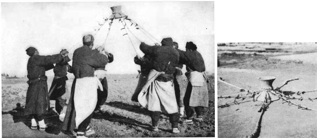
Figure 5.11 The two photos show the traditional way of compacting soil using stone flappers. This was introduced in the last chapter; the technique was still in use in the early twentieth century. Source: Todd, p. 7.
