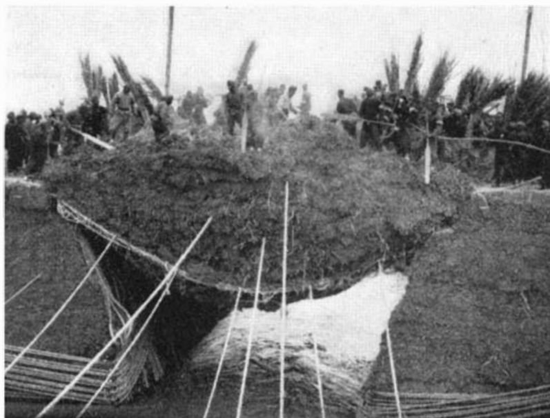
Figure 5.6 Another photo shows a kaoliang work being placed into the water. Source: Todd, p. 9.
