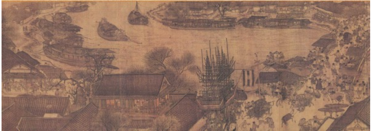
Figure 2. 21 Part of the painting Along the River During the Qingming Festival shows a busy scene along the Canal in Kai Feng, and the type of canal boats that were used during this period, as well as a boat being built on the bank. The earth embankment and trees can be also seen. There are arguments about the species of the trees in the painting as some are hard to recognize. Zhu and Xue believe that the two big trees in the middle might be Magnolia (left) and locust tree (right). 262 Source: Unknown, ‘quan juan qing ming shang he tu (the full length Along the River During the Qingming Festival )’, China Lizhi Website (2016) < http://www.zhlzw.com/lz/yis/793213.html > [accessed 30 June 2016]
