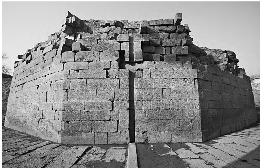
Figure 6.6 Another photo of the Tu Qiao Lock when it was discovered. The timber beams of the lock gate have gone, but the groove can be seen: 0.25-0.3m wide and 0.2-0.25m thick, and the detail of the stonework beside it. Source: Liao Cheng Institute of Cultural Relic Archeology, Liao Cheng Cultural Relic Bureau and Administration Office of Cultural Relic, Dong Chang District, Liao Cheng, p. 40.
