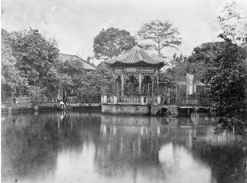
Figure 53 - VIEW B. “This gives you the ornamental water, the little summer house in the centre is where the friends of Hang How-qua retire to in hot weather to drink tea; I am upon the bridge leading to it, wh. is very rickety so I fancy it is seldom visited, the Inscription over the door on the board is Sow-chuck-qua wh. means I believe hot Flower house, the two Chinamen on the left are my servants whom I've drilled to sit steady, by going round where they are and looking back you see on the left and right No. 6 and 7.” John Frederick Crease. HP078416
