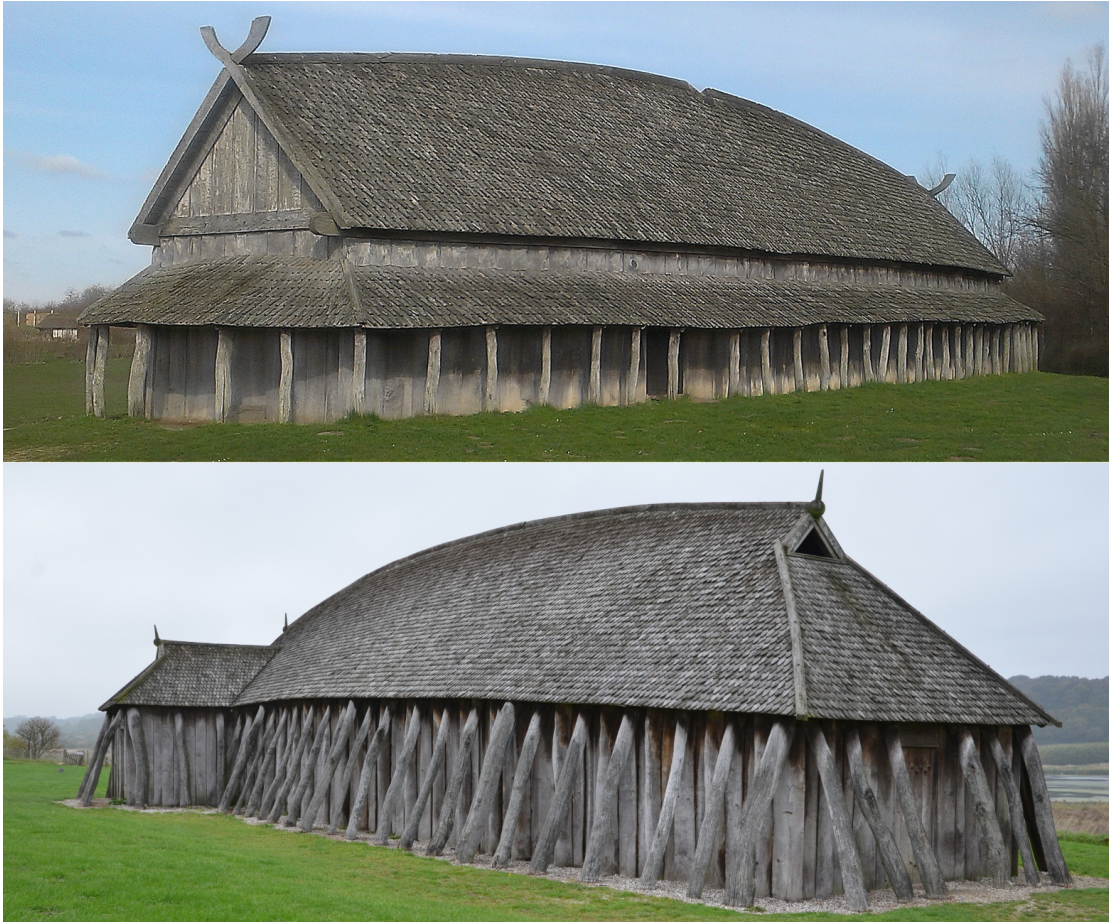
Figure 3.6: Photos of the reconstructed houses at Trelleborg (top) and Fyrkat (bottom). Photo: Anne Pedersen (top), Peter Jensen (bottom).
