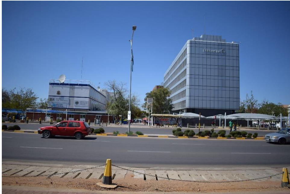
Figure 4.16: Newly refurbished buildings are dressed in aluminium cladding (source: taken by author in Gaborone 2016)
