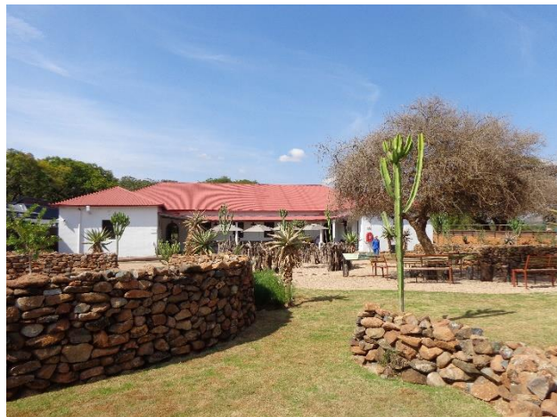
Figure 6.20: The walls are built to portray an impression of a dry stone traditional wall construction (Source: Nabeel Essa)
