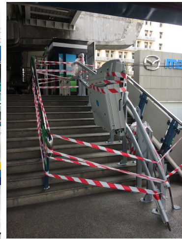
Image 2. Stair-lift at BTS
