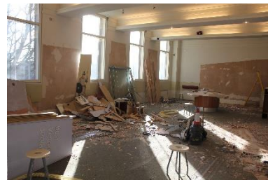
Figure 18. February 2016 – De-install of History Lab
