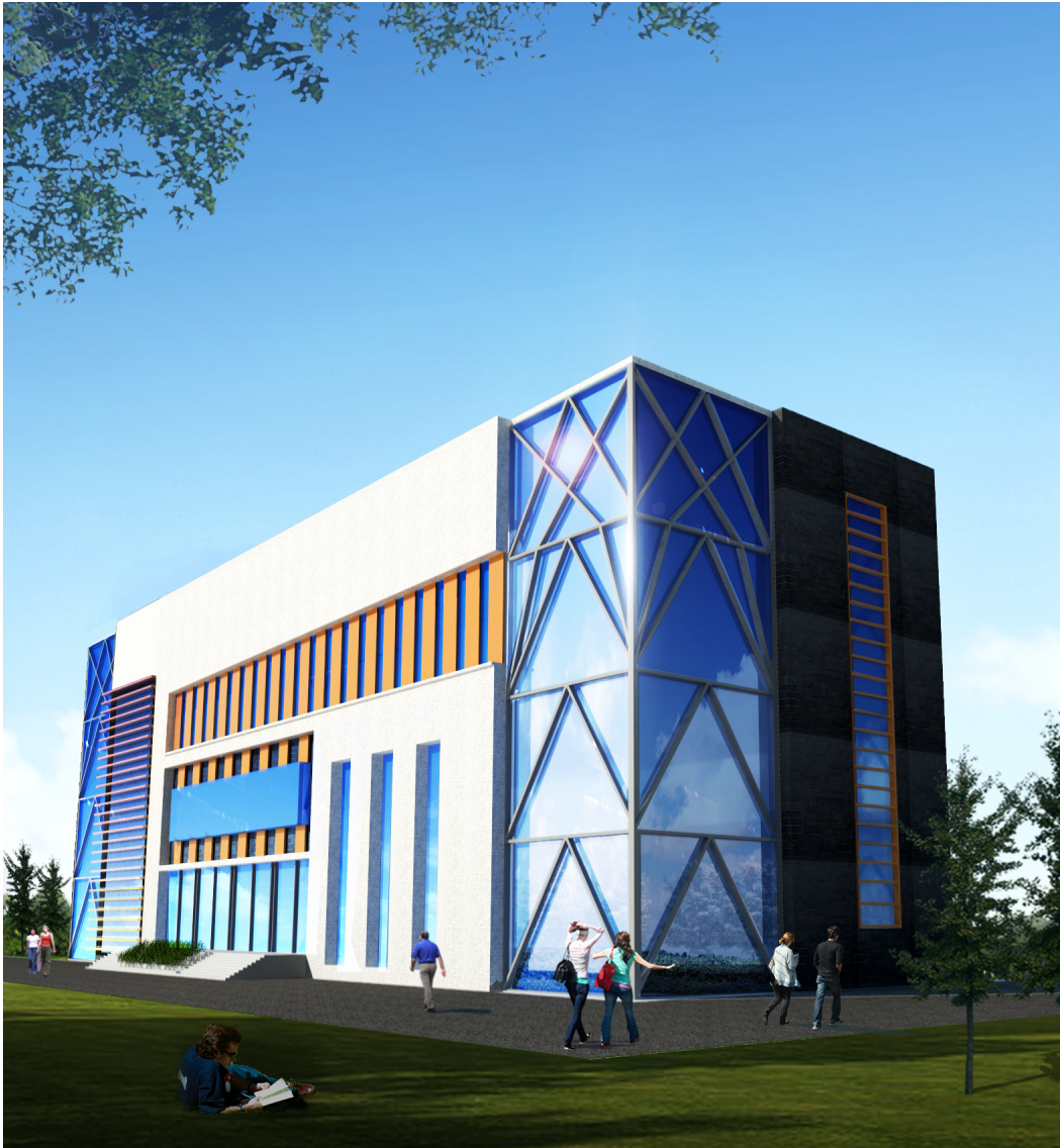
Figure 5.8: Visualization of small office building employing optimized bracing structure shown in Fig. 5.7b
