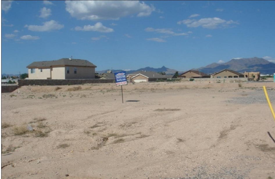
Figure 7.2 (a): Photograph of rilling due to water erosion on the lot cleared for housing developments in the East Mesa
