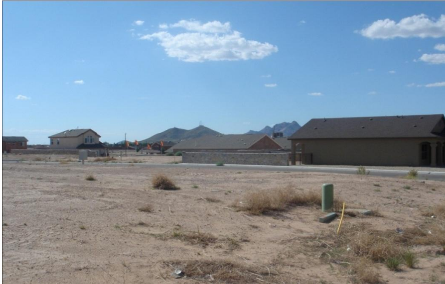
Figure 7.1 (a): Photograph of cleared lot for new developments in the East Mesa
