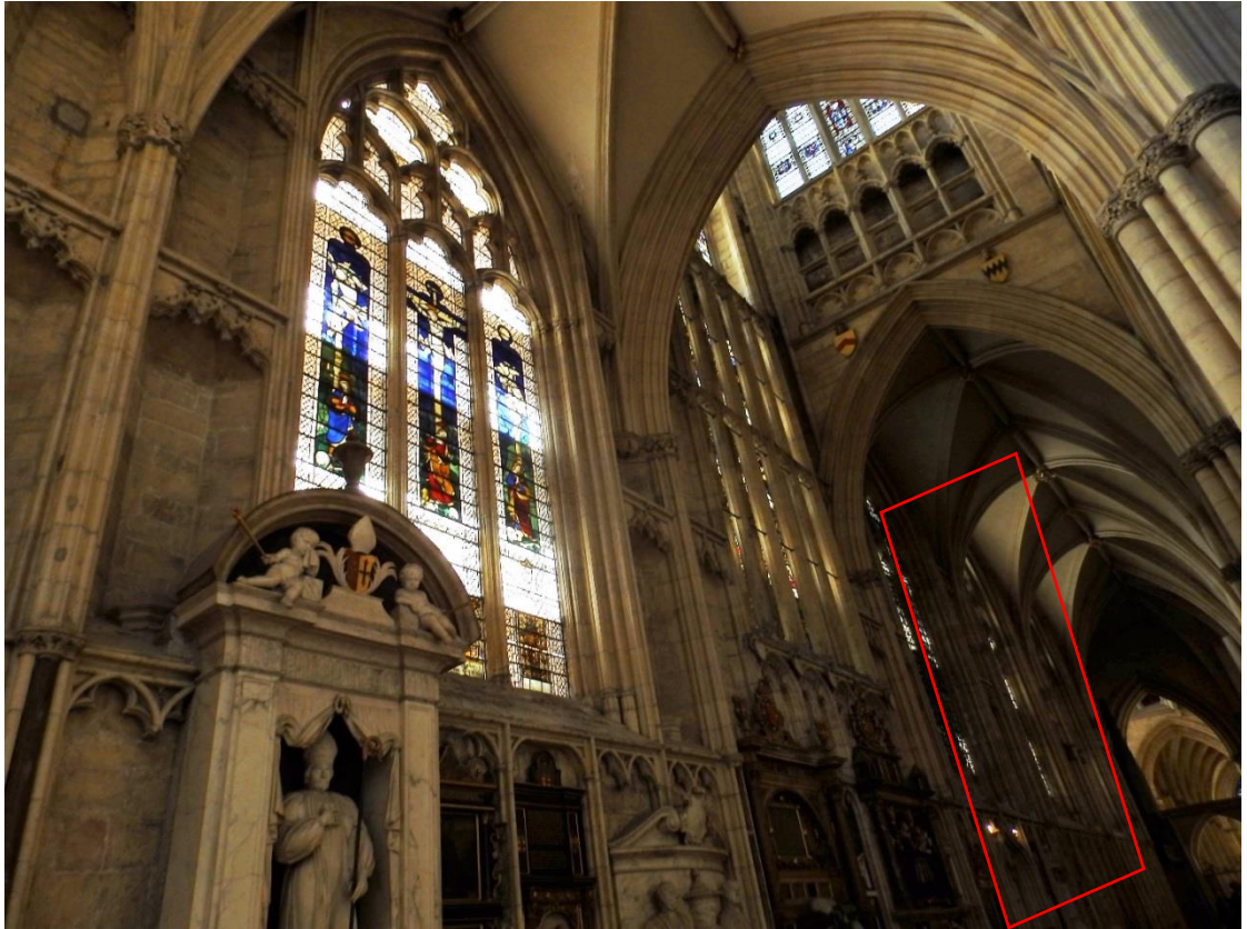
Figure 52: The south quire aisle looking west.
