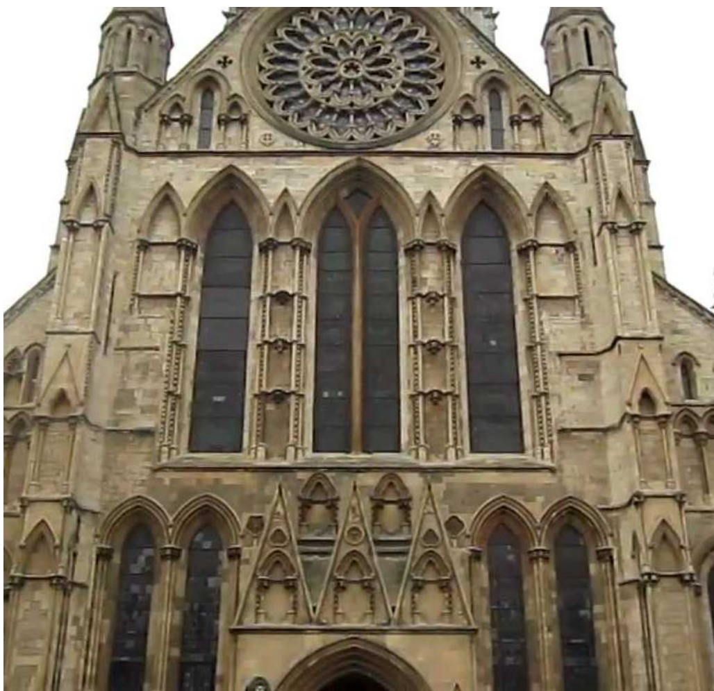
Figure 12: The central section of the southern façade.
