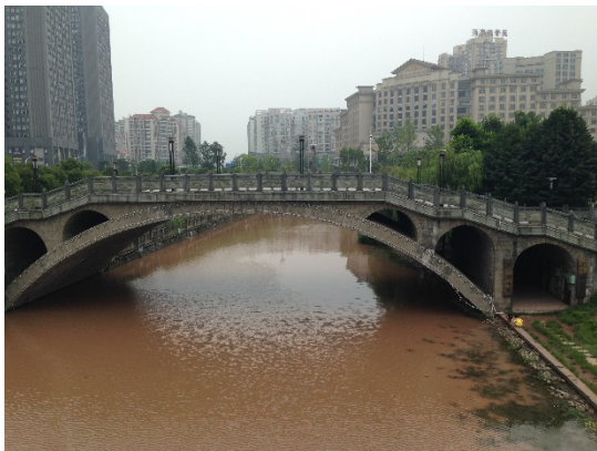
Figure 5-22 Bridges at the entrance of the square
