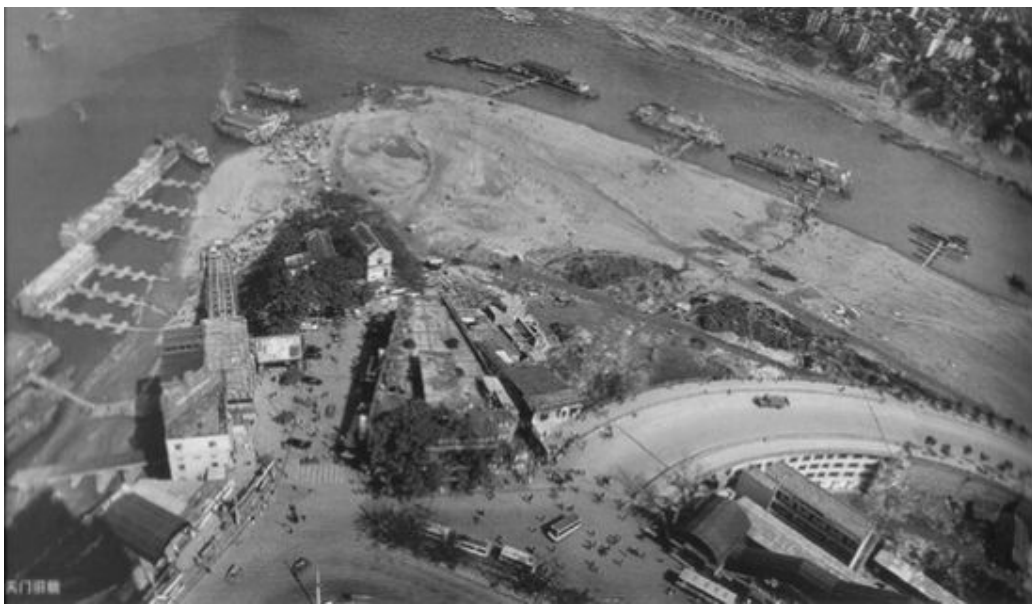
Figure 5-2 Chaotianmen wharf before the square was built
