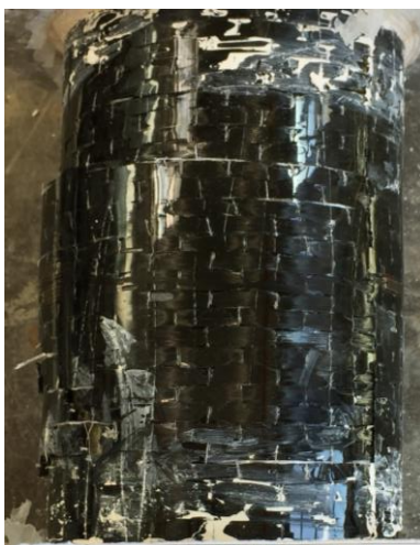
Figure G.93 Photos of 2C-C3
