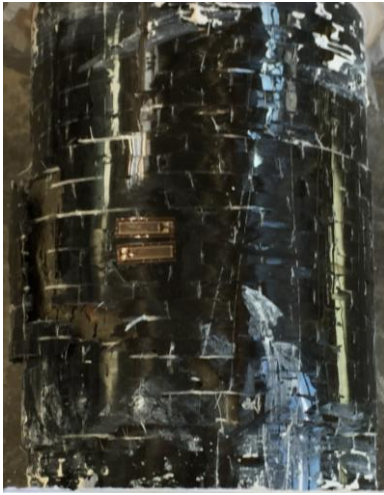
Figure G.95 Photos of 2C-C3
