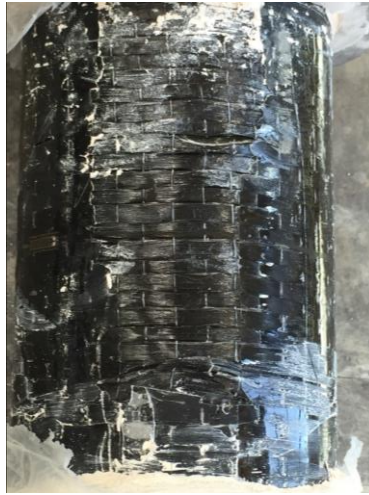
Figure G.96 Photos of 3C-C3
