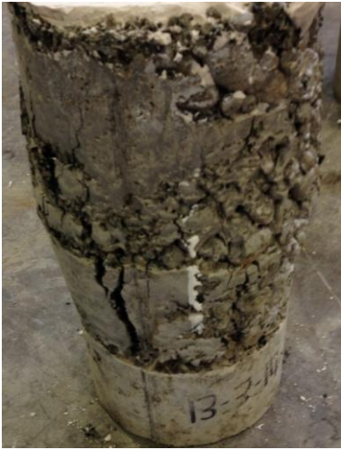
Figure G.9 Failure of mix O4
