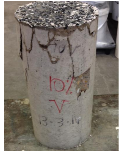
Figure G.3 Failure of mix O2
