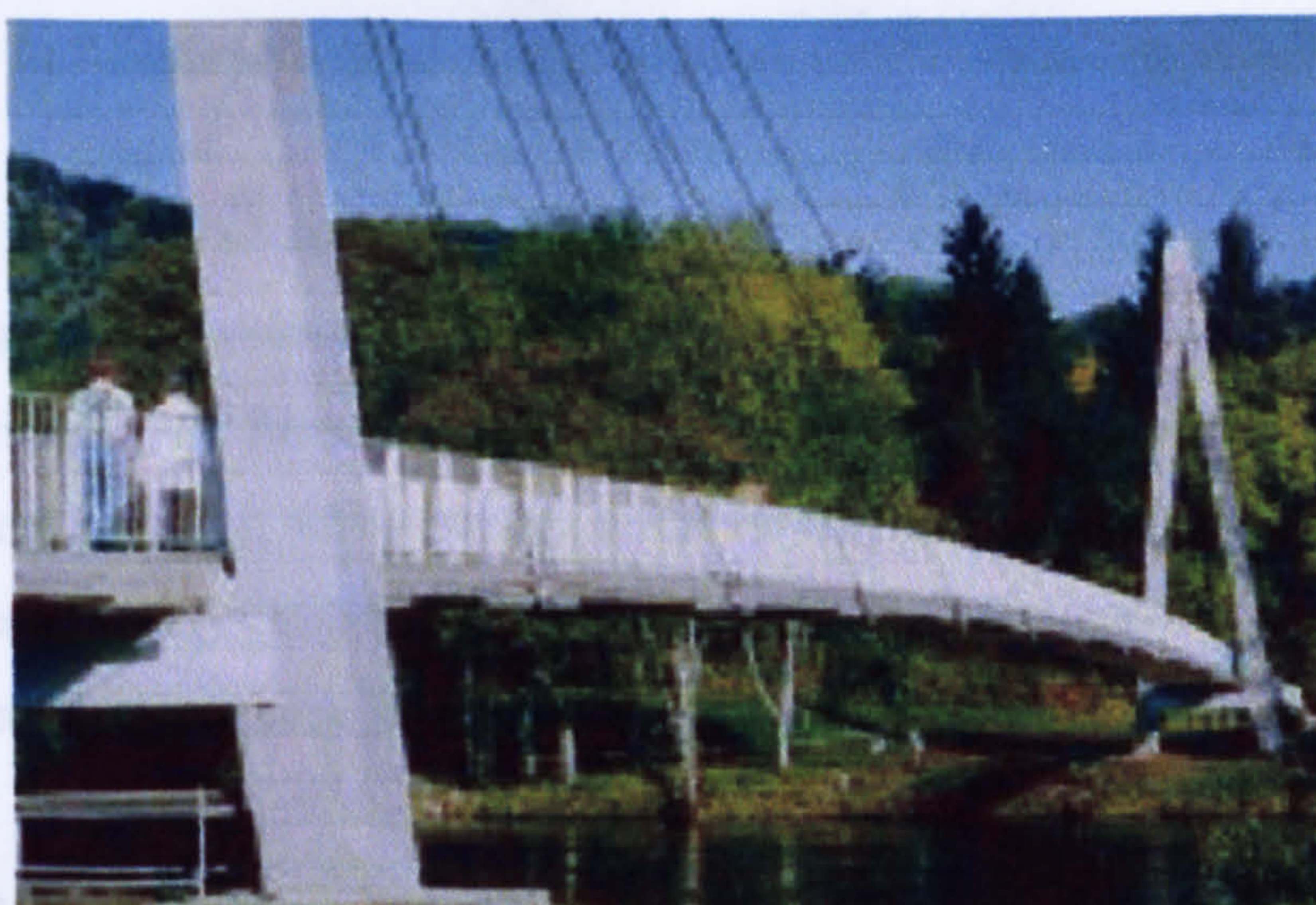
Plate 1.3 The Aberfeldy golfers' motorised bridge. Example of a structure made entirely from composites, Aberfeldy, Scotland, UK (After Burgoyne and Head, 1993)
