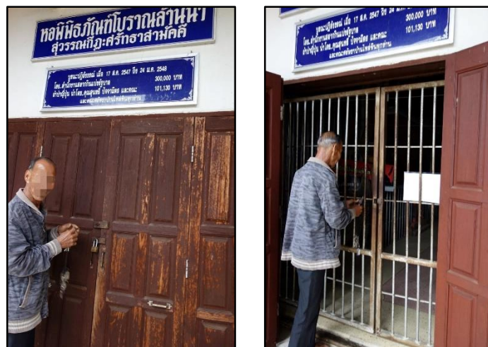
Figure 4.42: Double-layer secured wooden and iron gate with padlock, monastery museum, Wat Laihin, Lampang
