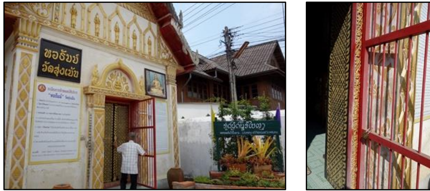
Figure 4.41: Double-layer secured wooden gate with padlock, Library of Palm Leaf Scriptures, Wat Sungmen, Phare
