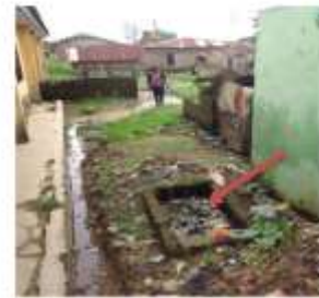
Open pit located near a path and receiving sewage
