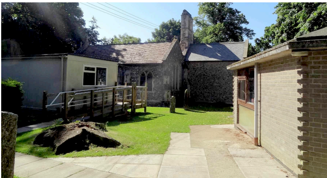
Fig. 4: Church of St Laurence, Brundall – view from north with Rainbow Room to left and Church Room to right
