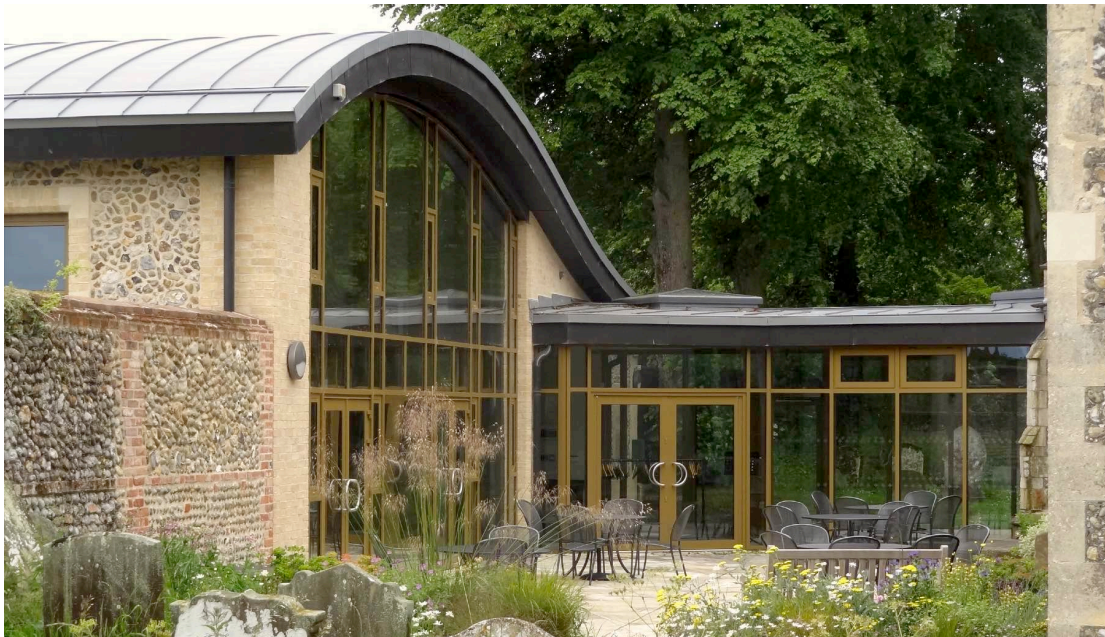
Fig. 7: Church of St Andrew, Holt – view of courtyard from east with churchyard wall to left
