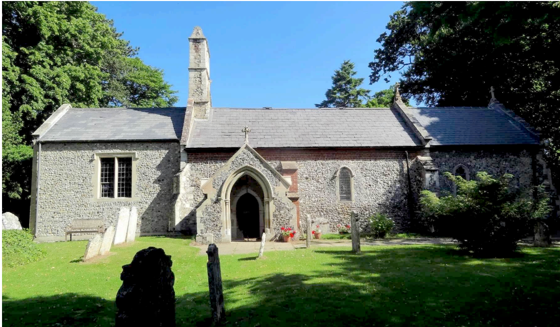
Fig. 3: Church of St Laurence, Brundall – view from south
