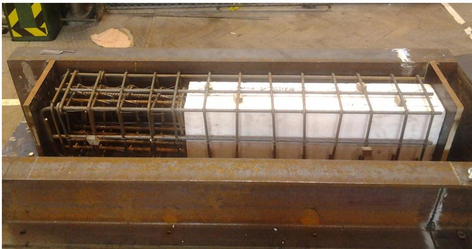
**Figure 3-13 Reinforcement cage of the precast U-beam**
