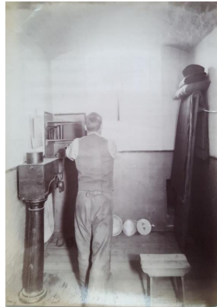
Figure 2.6 Hand crank at Wormwood Scrubs
