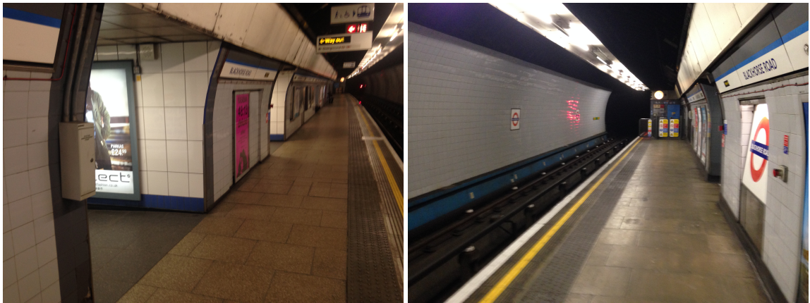
(a) The northbound platform looking south.
