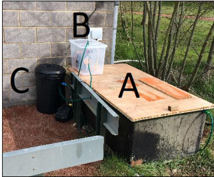
Figure 5.2.1.4. Pilot system buffer tank, delivery and discharge hydraulics. A = buffer tank; B = Prominent Delta delivery pump (to duckweed tank 1); and C = discharge trap containing submersible pump.
