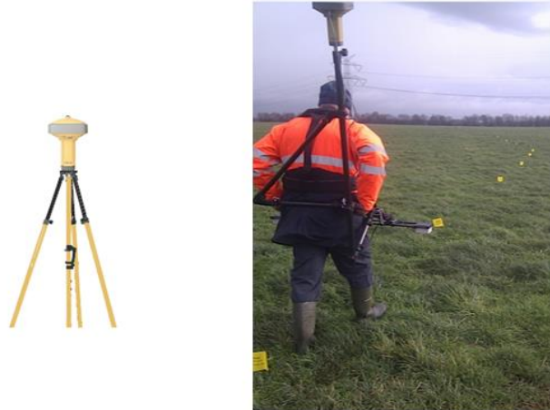
Figure 7.3: GR5 base station (left) and following pipe line route (right)
