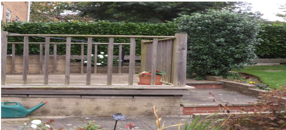
Figure 6.5 Private back garden with ramps, steps and rail for inclusive access.
