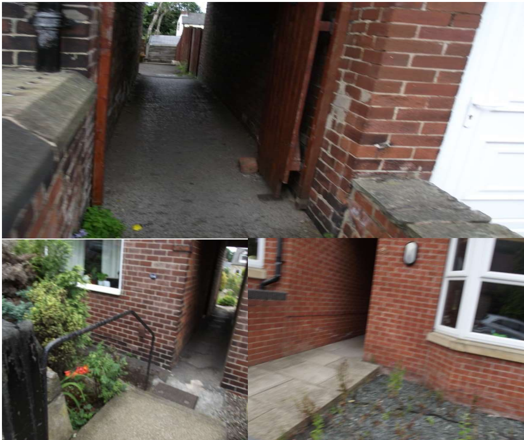
Figure 4.27 Some alley ways in terraced housing in Walkley Neighbourhood, Sheffield. (Source: Author's field Survey, 2016)
