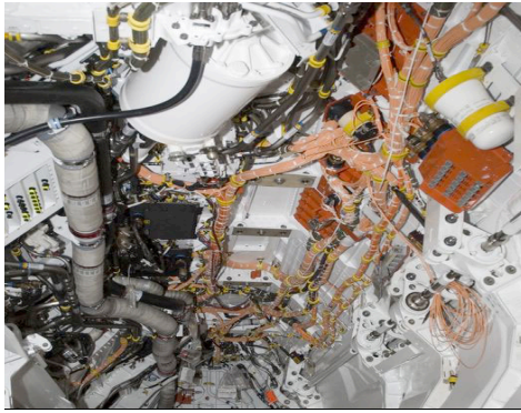
Figure 1.1: Some of the 20km of wiring on the JSF
