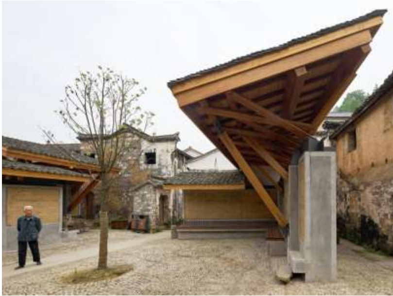
Fig. 6.23 Two new pavilions in single pitch tiled roof provide seating area and reorganize the communal square adjacent to the village ancestral hall. (Photograph by Zheng Shi)
