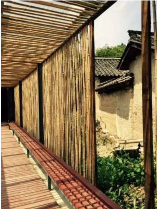
Fig. 4.10 A light-weight corridor connects the community hall and the mini-museum, and provides a linear space under the eave to enclose the public square in between. Summer 2015 (Photograph by Wei He)
