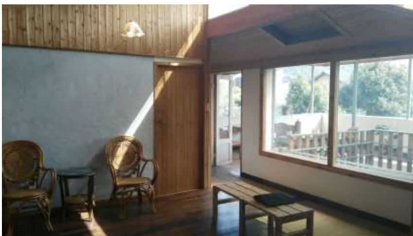
Fig. 8.30-31 Open plan of the first floor of Lodge No.1 with timber cladding on the earth wall. Top-lit corridor was wrapped by wood plate but still allowed enough natural light from the side parts. An enclosed bedroom, a bedroom- lounge, and a study room with good view connection with the semi-outdoor roof-top tea house. (Photograph by the author)
