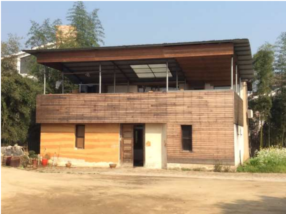
Fig. 8.10 External view of Lodge No.1 after refurbishment in 2015. (Photograph by the author)
