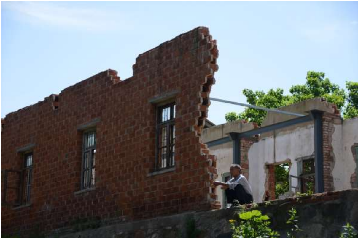
Fig. 4.16 Construction process of canteen. Summer 2014 (Photograph by Wei He)
