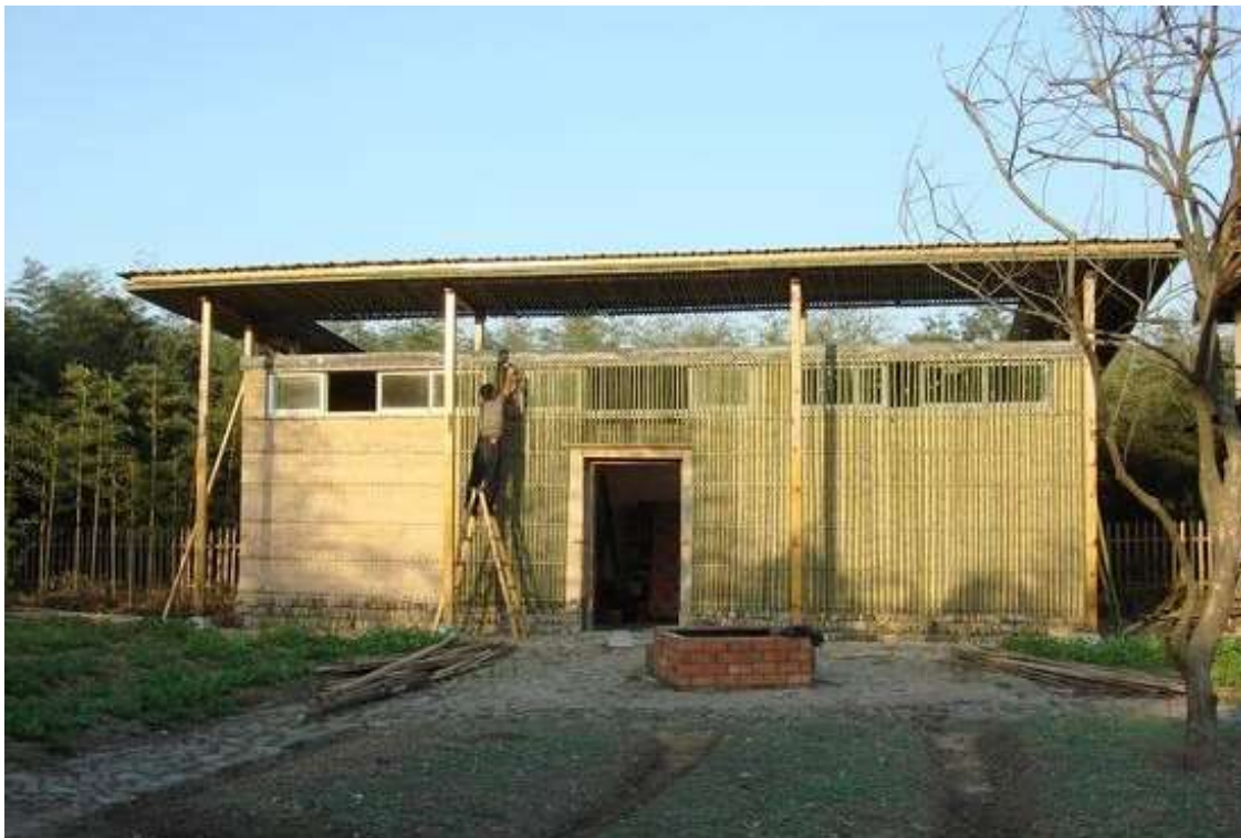
Fig. 8.41 The first refurbishment of Lodge No.4 in 2007 introduced a bamboo canopy and claddings onto the rammed-earth free-standing walls and the pre-cast concrete roof. (Photograph by Weizhong Ren)
