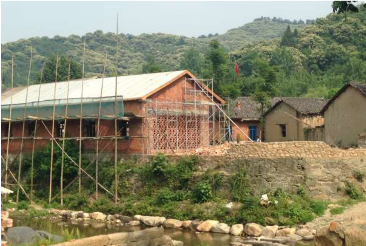
Fig. 4.17 Construction process of canteen. Summer 2014 (Photograph by Wei He)
