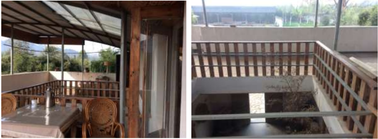
Fig. 8.28-29 The later-added metal roof supported by light-weight steel tubes, provided a semi-outdoor space for tea house and a bathroom. A PV panel and a wooden balustrade were also installed to protect the courtyard. (Photograph by the author)
