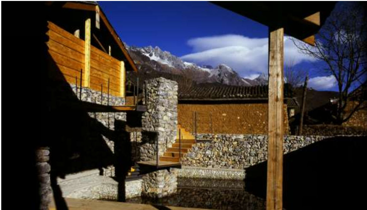
Fig. 3.27 The 'Elementary School Expansion' done by Li Xiaodong Atelier in Yuhu village, Yunnan province. (Photograph by Xiaodong Li)
