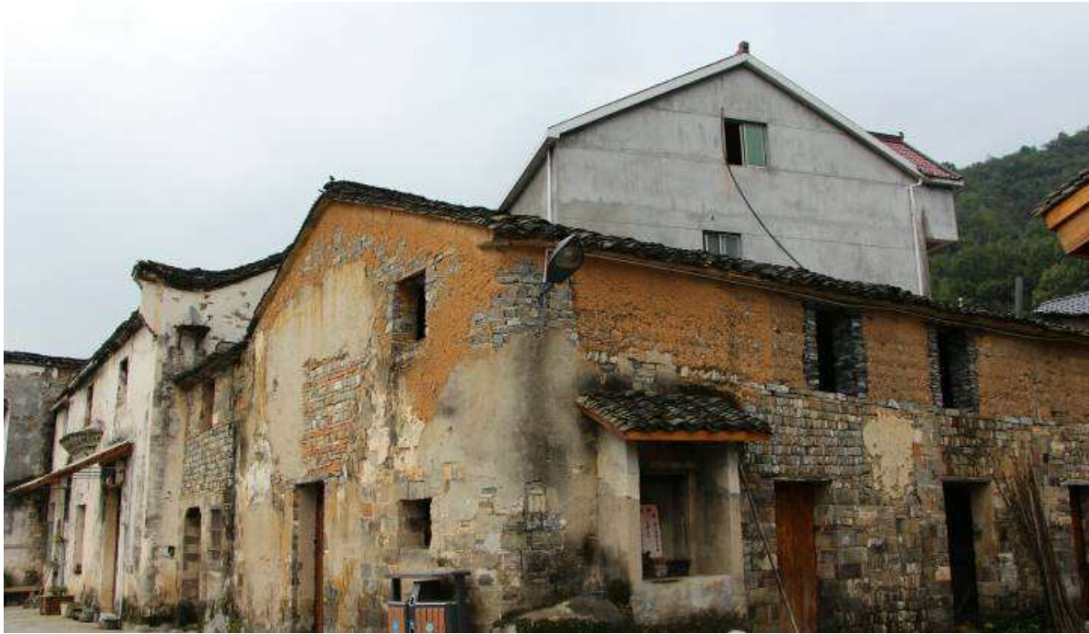
Fig. 6.7 For architecture without architects in Wen village, the building object is not only a provisional assemblage of numerous materials ranging from earth to pebbles, but also a constant building process that is socially constructed through many hands and heads. At the back of this messy-engaged building is a new apartment in much 'cleaner' method and appearance. (Photograph by the author)
