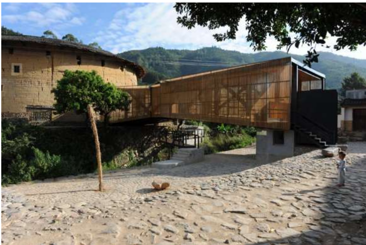
Fig. 3.28 The 'School Bridge' done by Li Xiaodong Atelier in Xiashi village, Fujian province. (Photograph by Xiaodong Li)
