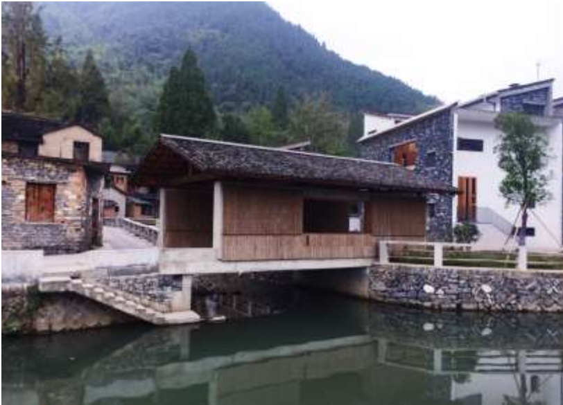
Fig. 6.17 A rain-water bridge in concrete load-bearing walls and wooden roof is placed at the intersection between new housing part, old village, and the river, marking a communal focal point for the village. (Photograph by the author)
