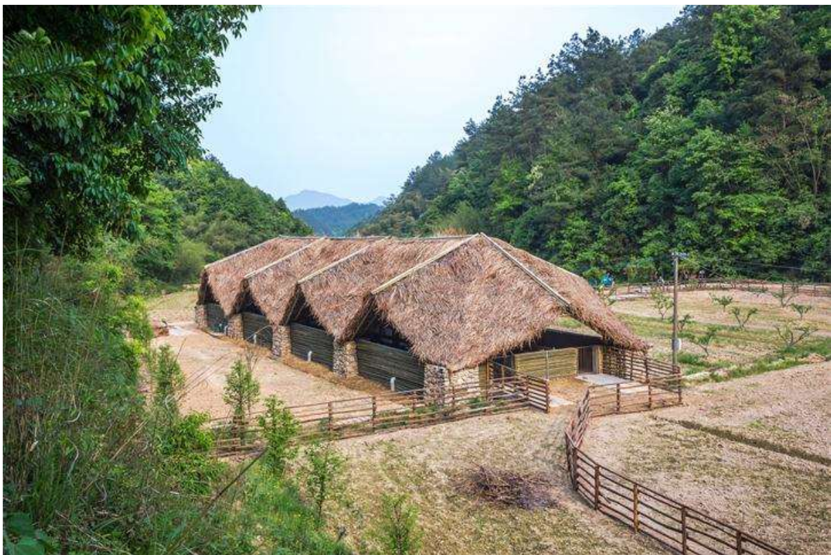
Fig. 5.1 The pig barn of ‘Sun Commune’ in Shuangmiao village (Photograph by CITIARC)
