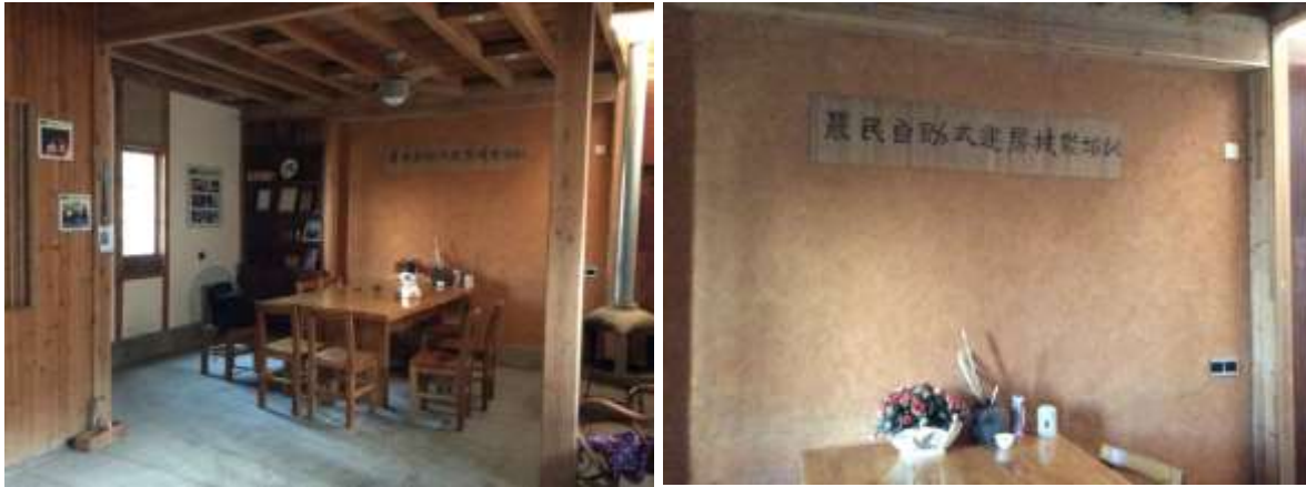
Fig. 8.14-15 The rammed earth and timber structure worked side by side in the multi-functional hall at the ground floor of Lodge No.1. (left): a welcoming space with screen as exhibition wall, and a meeting/dining space; (right): the tablet on the wall showing its aspiration as 'Rural Self-help House Design-build Training Centre'. (Photograph by the author)
