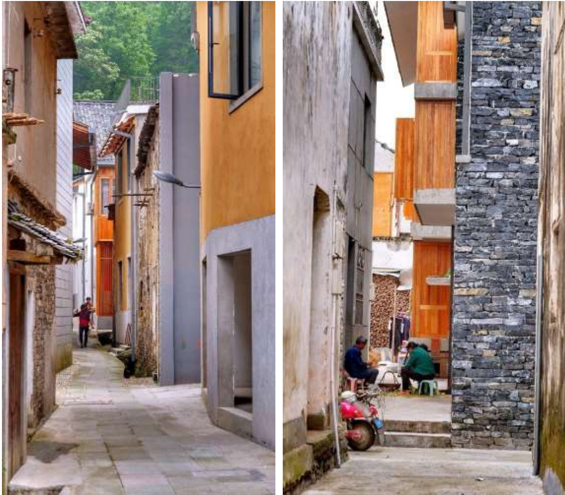
Fig. 6.25-26 The interface between the new added and the old existing inside Wen village (Photograph by the author)
