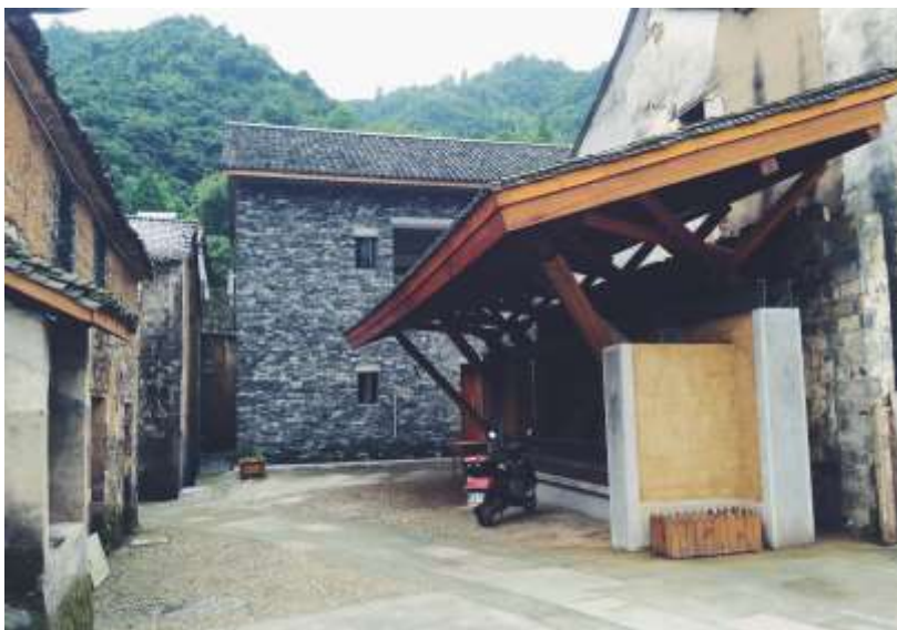
Fig. 6.24 Another resting pavilion provides a shared space under the eave for a small piazza (Photograph by the author)
