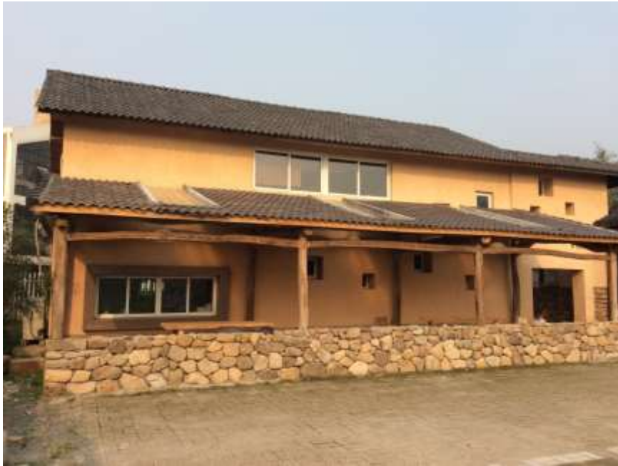
Fig. 8.43 External view of the fifth lodge in 2015. (Photograph by the author)
