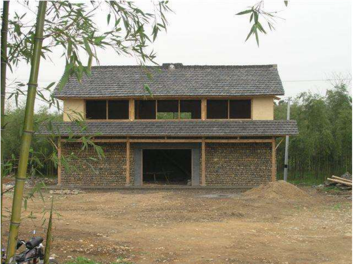
Fig. 8.32 Lodge No.2 in 2007, after the assembly of the main structure recycled from old buildings. A strong frontality borrowed from traditional typology of ancestral halls. (Photograph by Weizhong Ren)
