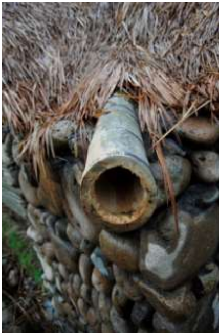
Fig. 5.18-19 The drainage pipe made of bamboo directed rainwater from the thatched roof to the pebble foundation and finally returning back to the soil. (Left) (Source: Sun Commune); (Right) (Photograph by the author)
