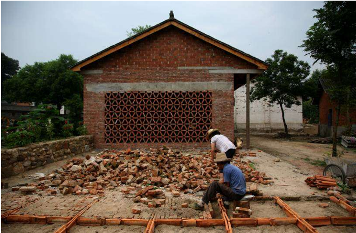
Fig. 4.15 Collective construction process on site. Summer 2014 (Photograph by Wei He)
