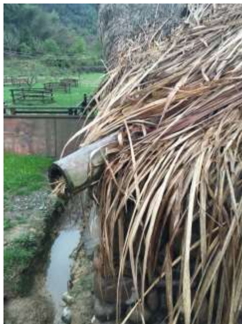
Fig. 5.18-19 The drainage pipe made of bamboo directed rainwater from the thatched roof to the pebble foundation and finally returning back to the soil. (Left) (Source: Sun Commune); (Right) (Photograph by the author)
