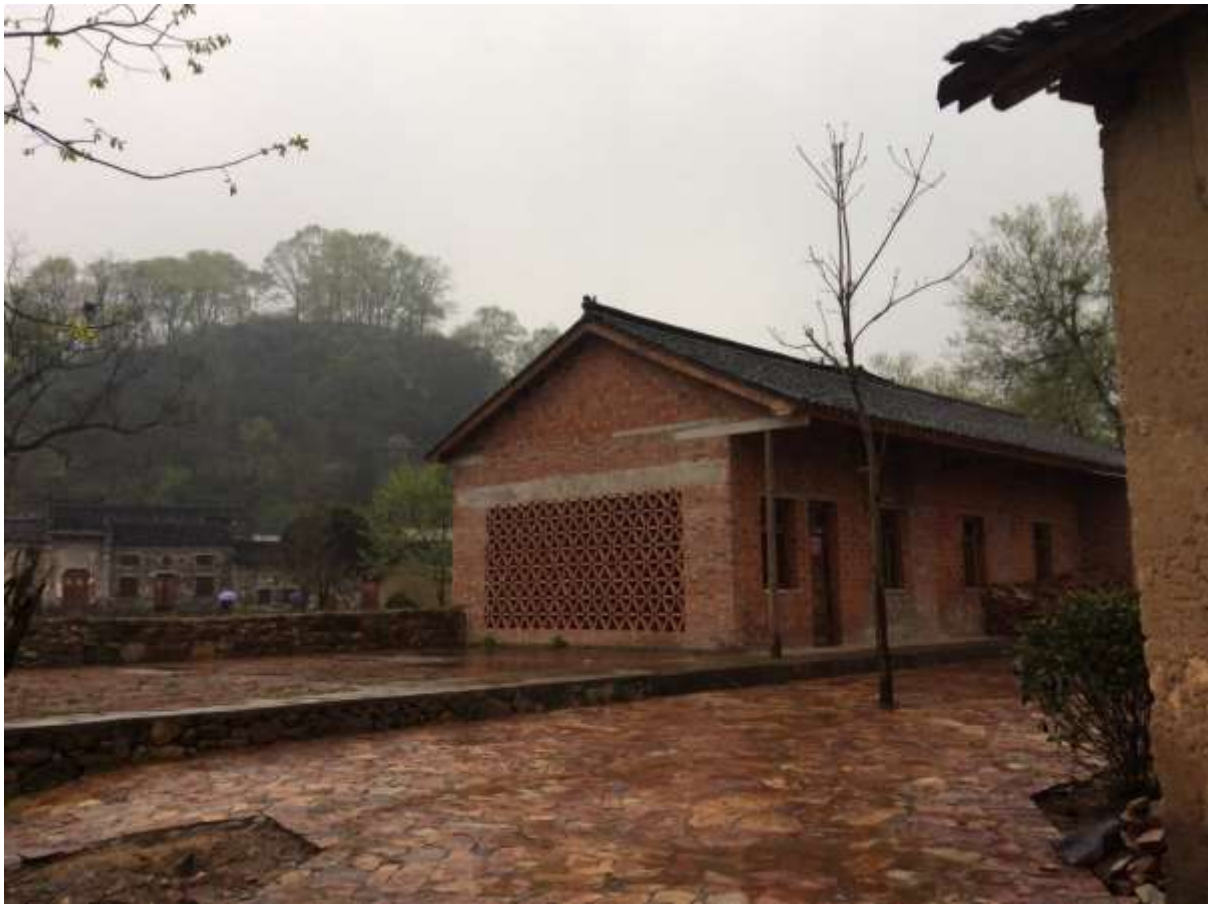
Fig. 4.12 A new canteen for the village was transformed from an abandoned building, with its external brick-screen-wall coproduced by the architect and users in a different way from both urban and rural normal practice. One third of the existing volume was demolished in order to leave a ritual visual corridor to assimilate Qi (energy) to the main body of the village on the other side of the river. Spring 2015 (Photograph by the author)
