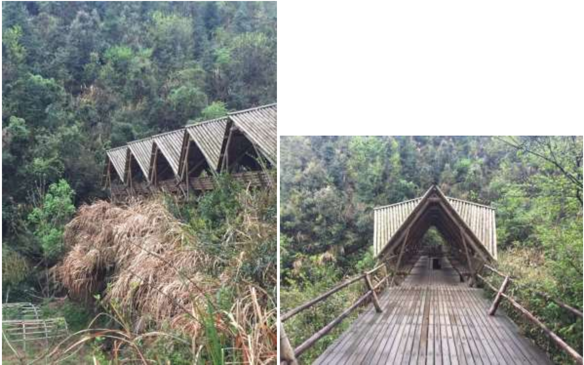
Fig. 5.24-25 In the second phase of 'Sun Commune', a semi-outside structure with five spatial units using similar design methodology with the pig barn was built upon the wildness, functioning both as footbridge and a tea house. It restored and reinvented the old memories of Wind-rain-bridge in traditional villages. (Photograph by the author)
