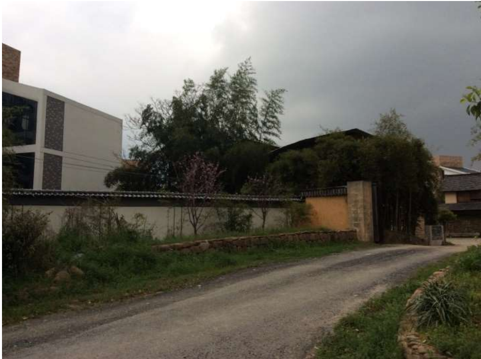
Fig. 8.8 The only gateway to Weizhong Ren's site of Eco-Lodges. One of the newly developed villa clusters was only divided by a small bunch of bamboo with Ren's lodge. It shows a Chinese-characteristic 'handshaking building' phenomenon. (Photograph by the author)
