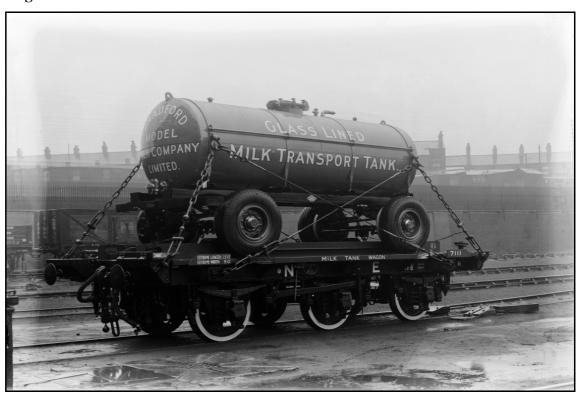
Bradford Model Milk Company Limited 2,000-gallon demountable milk tank and flat-wagon, illustrating the arrangement pioneered by the Southern Railway and the London Cooperative Wholesale Society at the latter's Bruton dairy in 1931. Although undated, the wagon was probably constructed by the LNER c1934. Source: National Railway Museum DS130202-101926.
