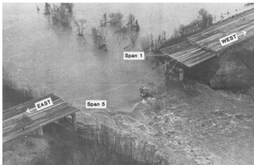
Figure 1.6: Aerial view of Schoharie Creek Bridge after failure (Swenson and Ingraffea, 1991).
