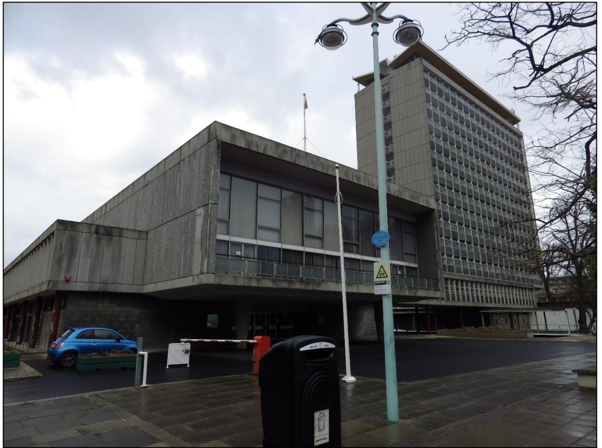
Figure 15 Plymouth Civic Centre, January 2016 (Source: © Martin Flook, 2016)
