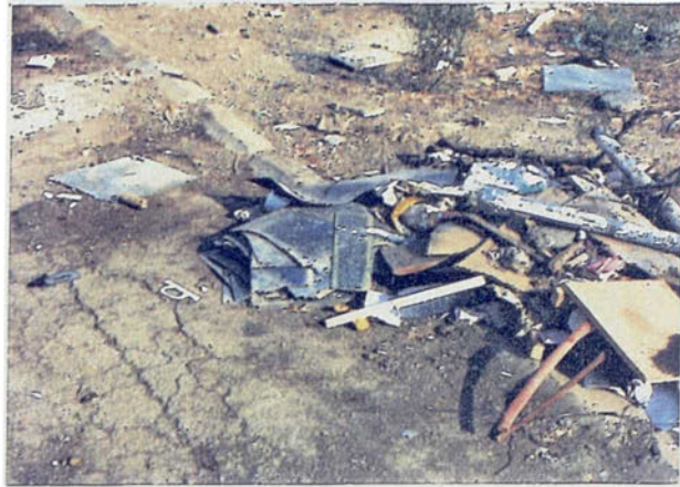
Figure 6.2 : Removal of the plastic doors and floor tiling
