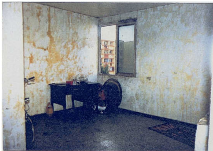
b. A veranda in the process of being closed off
