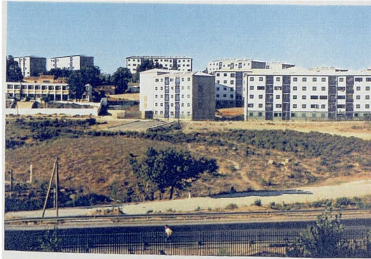
Figure 5.6 : Lack of hierarchy and definition of the external spaces in the Ain Allah estate
