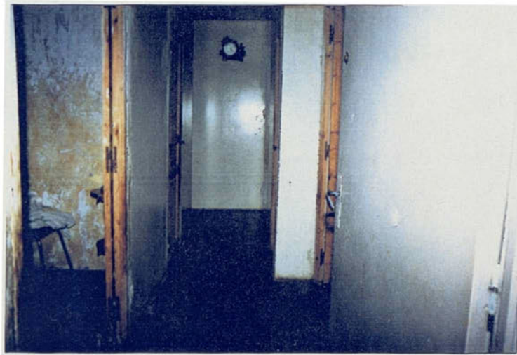
b. Replacement of the plastic doors by wooden doors and the plastic floor tiling by a ceramic floor tiling
