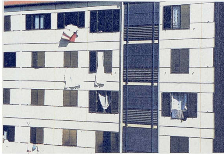
Figure 6.12 : Light prefabricated facade in the Ain Allah estate
