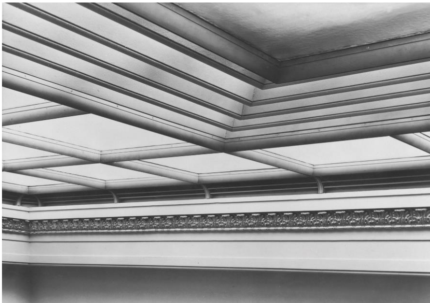
Figure 87. View of louvre laylights, National Gallery (1950) © Crown Copyright (NG30/1950/11; P6397_007)
