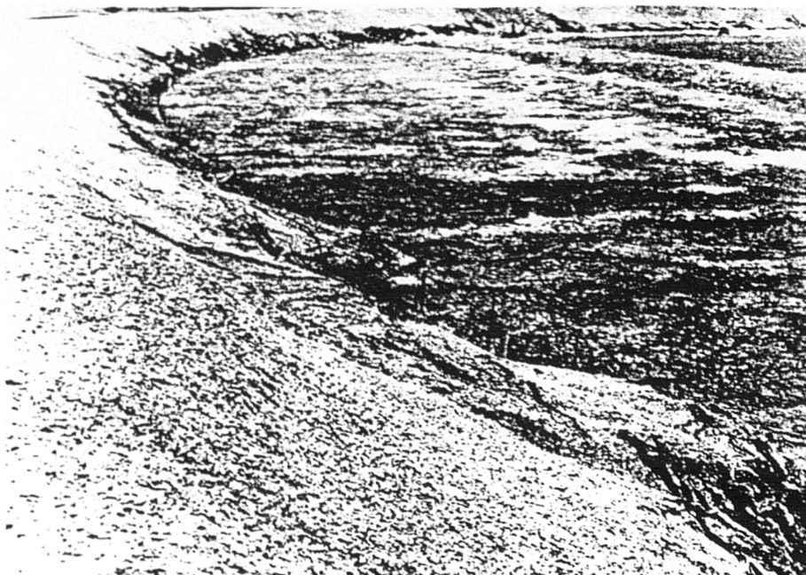
Fig. 1.4 : Failure of earth slope at Notch Hill, Canada due to wetting (Krahn, Fredlund and Klassen, 1989)
