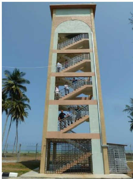
Figure 6.2. Image to show the atmospheric observation tower at the Bachok Marine and Atmospheric Research Station.
